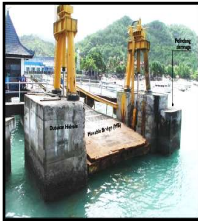
Sumber : Data OPP Lembar Gambar 4.16 Moavble Bridge Dermaga I
