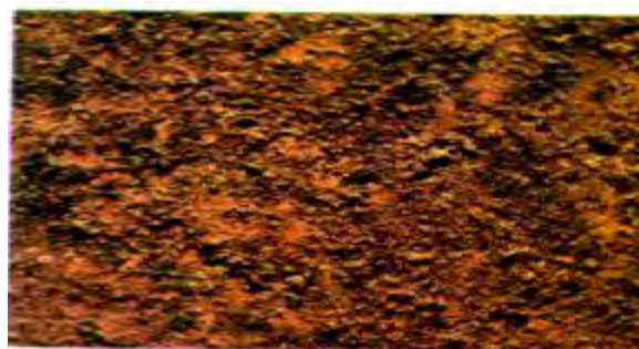
Gambar II.13 Rust Grade D (ISO 8501-1)
