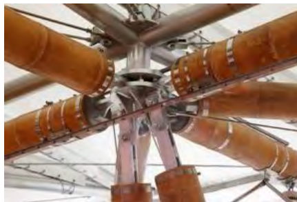
Gambar 2.12 Sambungan Modern Pan Knot
