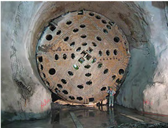
Gambar 5. 40 Tunnel Boring Machines
