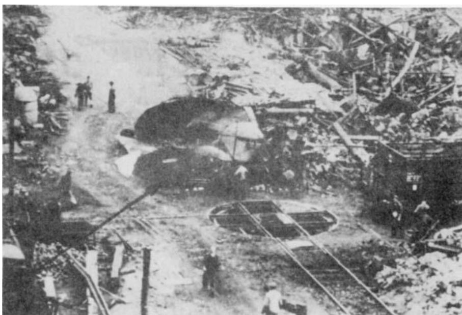
Figure 2.3. Port Hudson, Missouri disaster, this incident is resulted by vapor cloud explosion (CCPS, 1994). Source picture: CCPS Guidelines for Evaluating the Characteristics of Vapor Cloud Explosions, Flash Fires, and BLEVEs page 96
