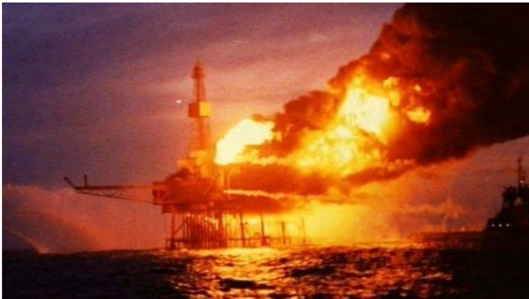
Figure 1.1. The Accident of Piper Alpha Explosion (BBC.uk, 2010)
