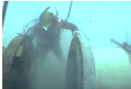
Gambar 2.8 Subsea Spool Installation
