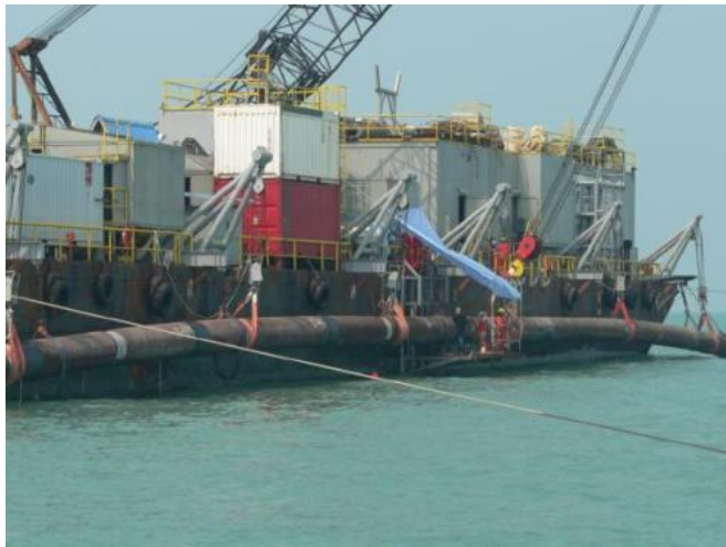
Gambar 2.9 Ilustrasi Above Water Tie-in ( irnhlsea.wordpress.com/2016/02/04/365/ )
