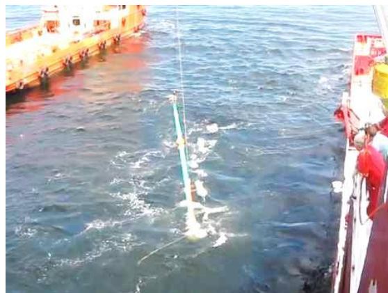
Gambar 2.6 Spool Lifting
