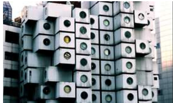
Gambar 5: Sistem Modular Nakagin Tower
