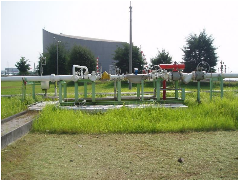
Figure 5.2 Meterring Station
