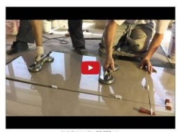
Instalasi ubin 60/120 cm
