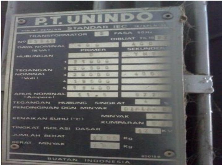
Gambar 9 Nameplate Transformator M.049-1
