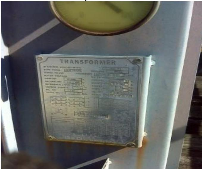
**Gambar 12** Nameplate Transformator M.180
