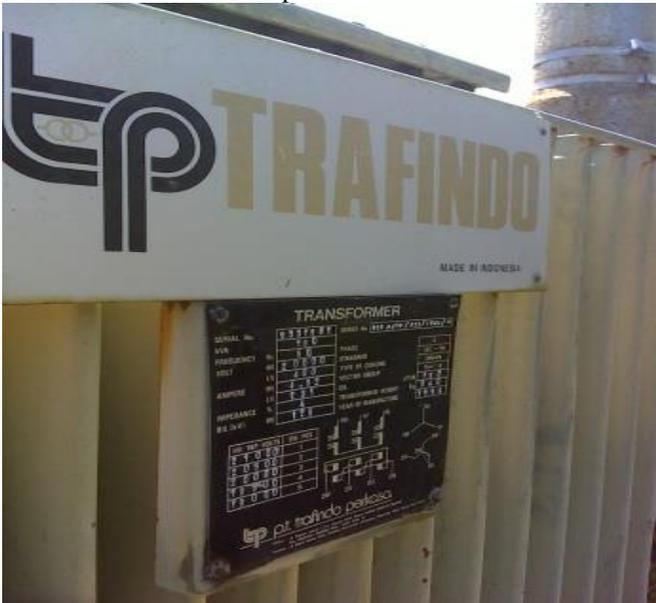
**Gambar 8** Nameplate Transformator M.040
