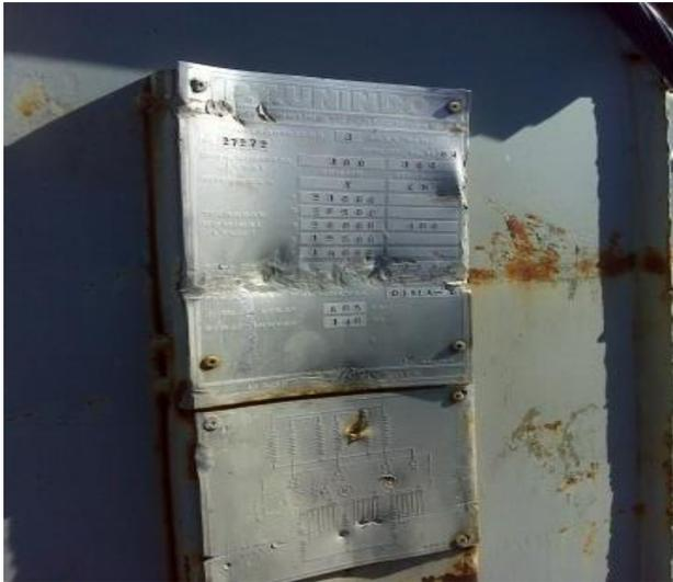
**Gambar 3** Nameplate Transformator M.218
