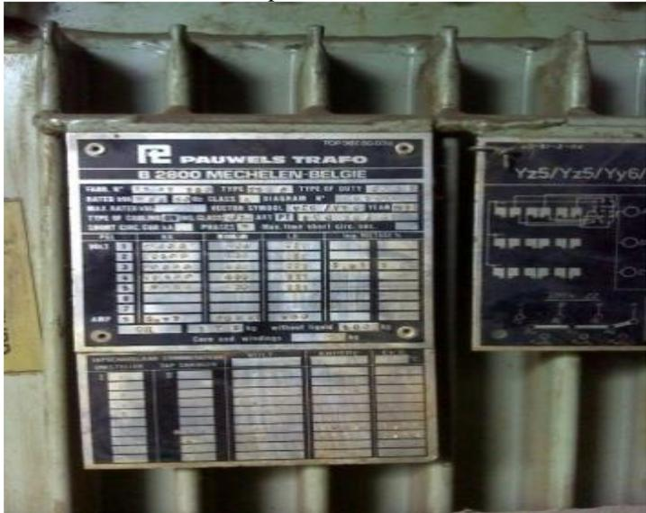
Gambar 10 Nameplate Transformator M.057
