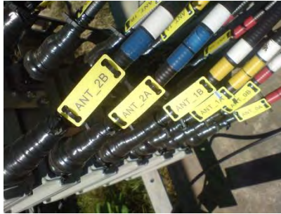
Gambar 3.5 Cincin Kabel Feeder BTS 2G
