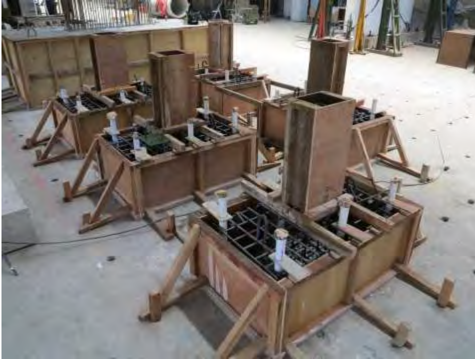
Figure 3-42 Prepared formworks and reinforcements of the specimens
