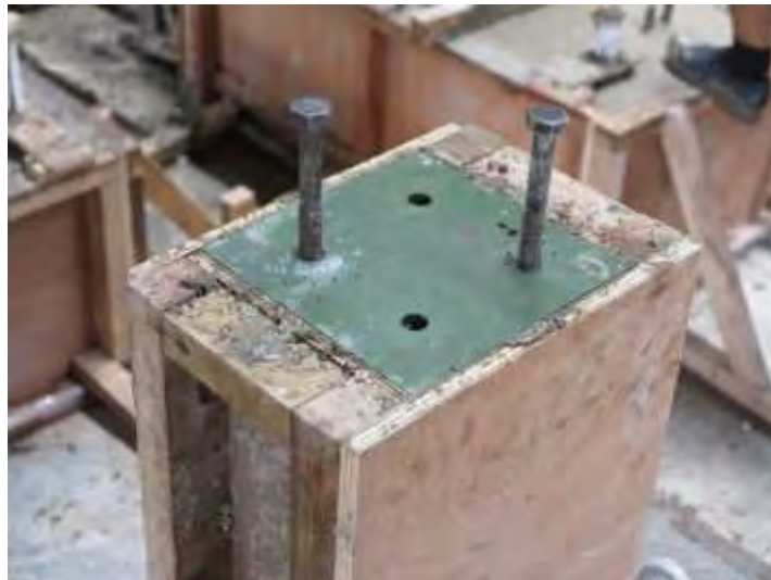
Figure 3-49 Steel plate of column head
