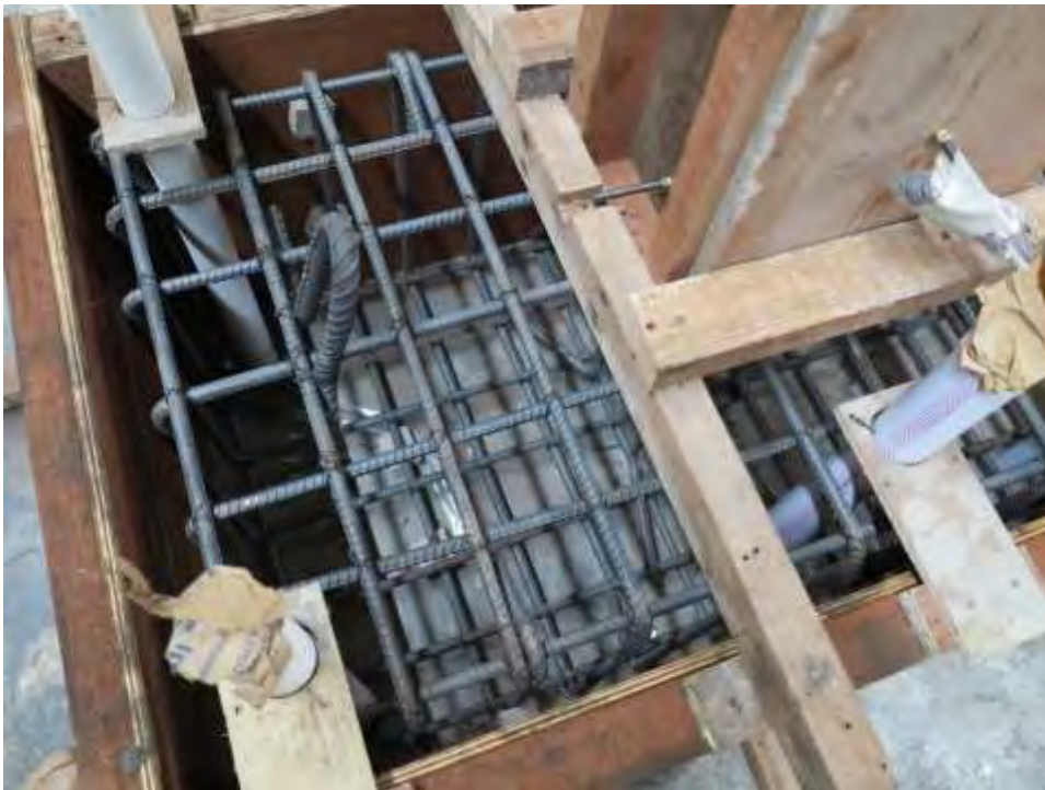
Figure 3-43 Reinforcement of typical footing of the specimens
