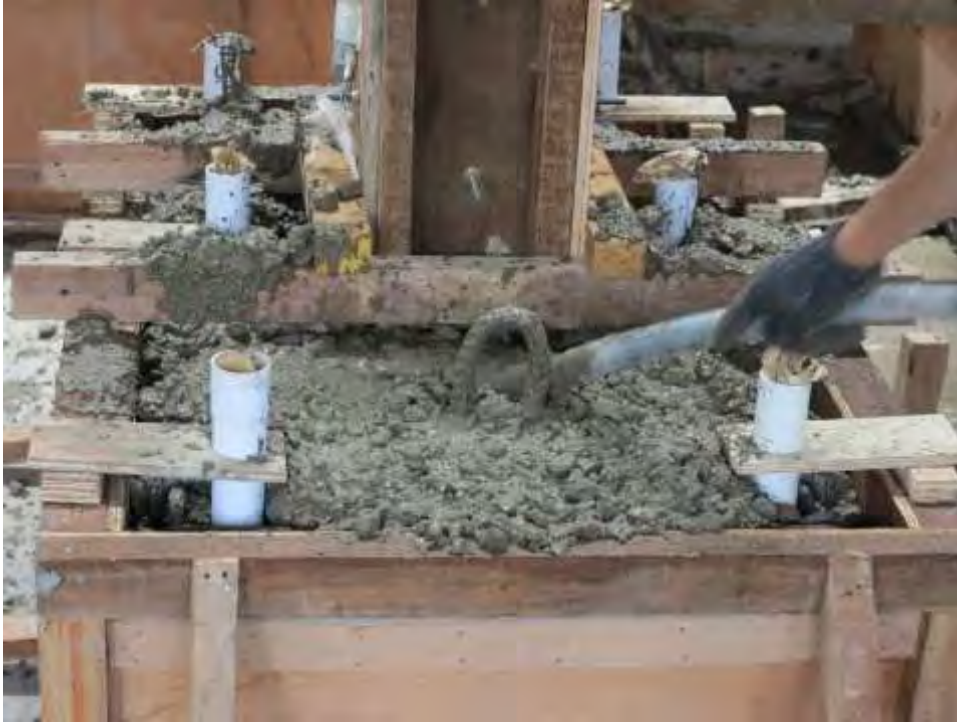
Figure 3-46 Concrete compacting of foundation
