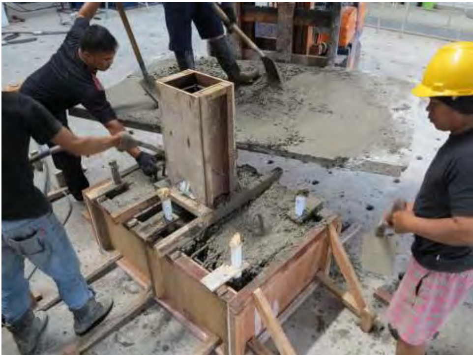
Figure 3-45 Concrete casting of foundation
