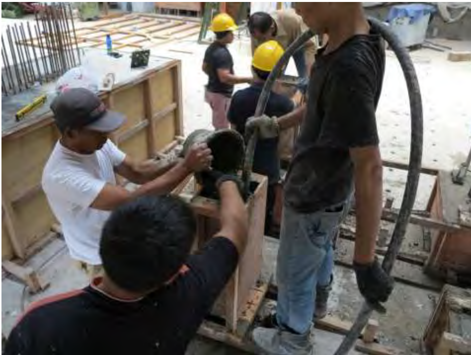
Figure 3-47 Concrete compacting of column
