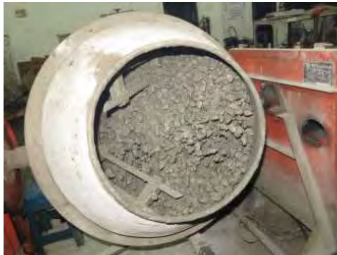
Figure 3-35 Concrete mixing process
