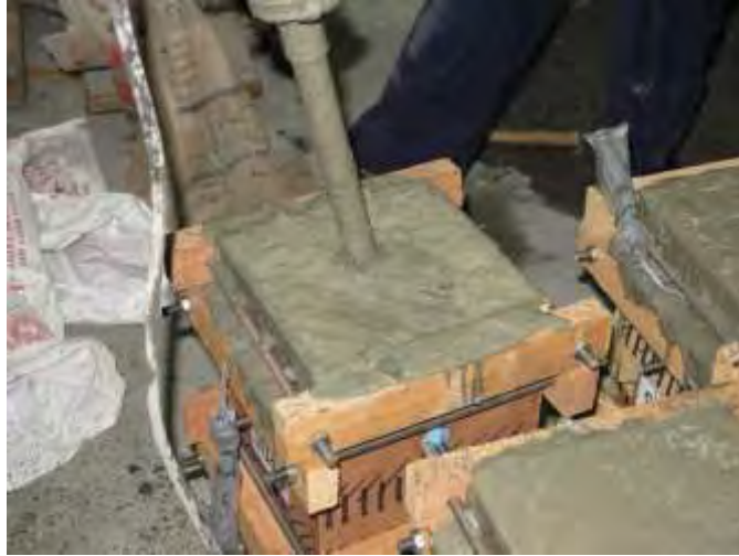
Figure 3-37 Vibrated concrete to minimize trapped bubbles
