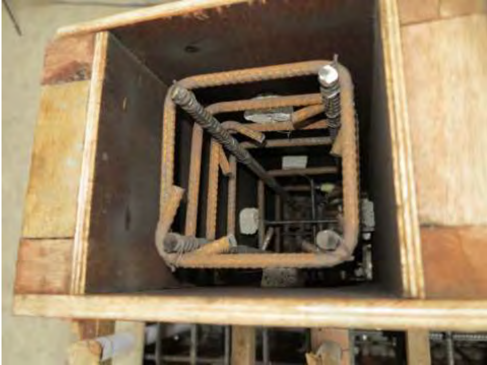
Figure 3-44 Reinforcement of column head
