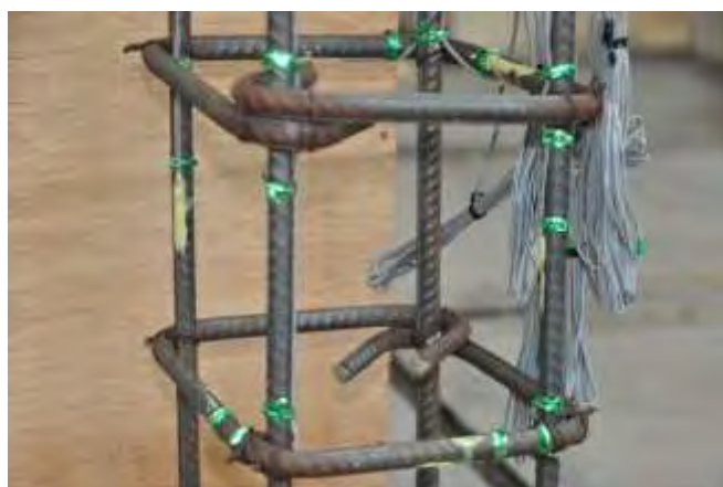
Figure 3-26 Typical placing of strain gauges on longitudinal and transversal bars in the test region
