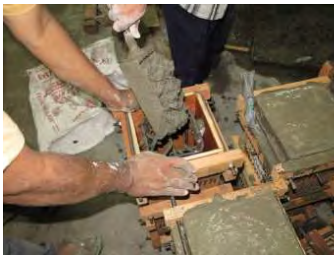
Figure 3-36 Concrete placing by using hand shovel
