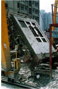
Gambar 4.7 Demoulding Dinding Pracetak
