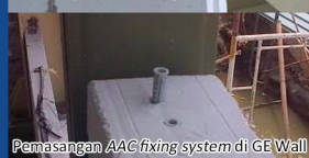
Pemasangan AAC fixing system di GE Wall
