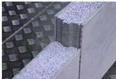
Gambar 4.19 Dinding Panel Beton Ringan
