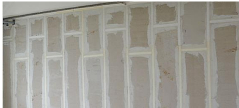
Gambar 4.23 Tampak Finishing Panel Terpasang
