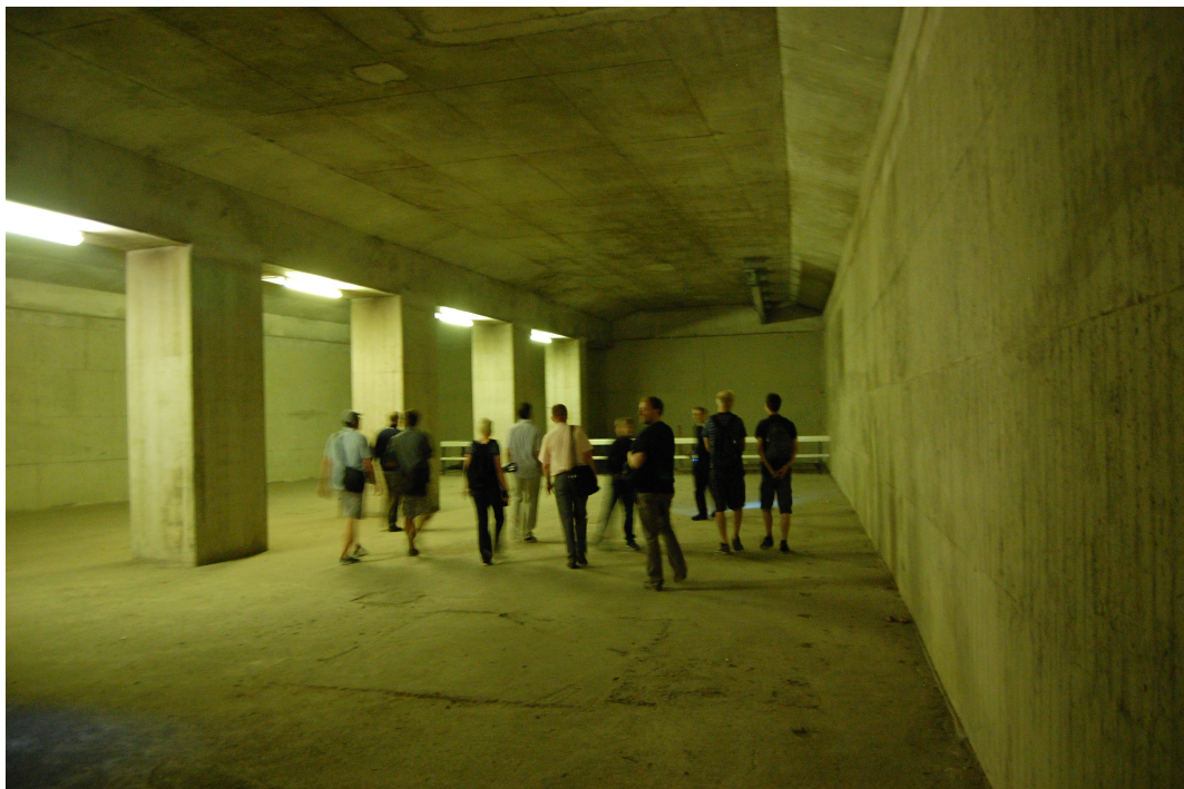
Figure 9.5. The incomplete U10 Innsbrucker Platz station. Source: Author 2013.
