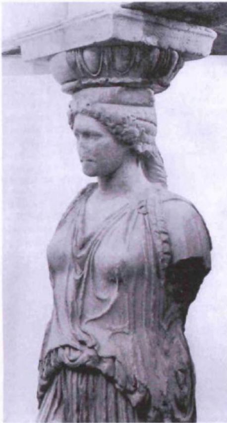
Figure 12a: view of a Caryatid, showing acid attack by acid rain on the front (source: Skoulikidis 1994b, 19).
