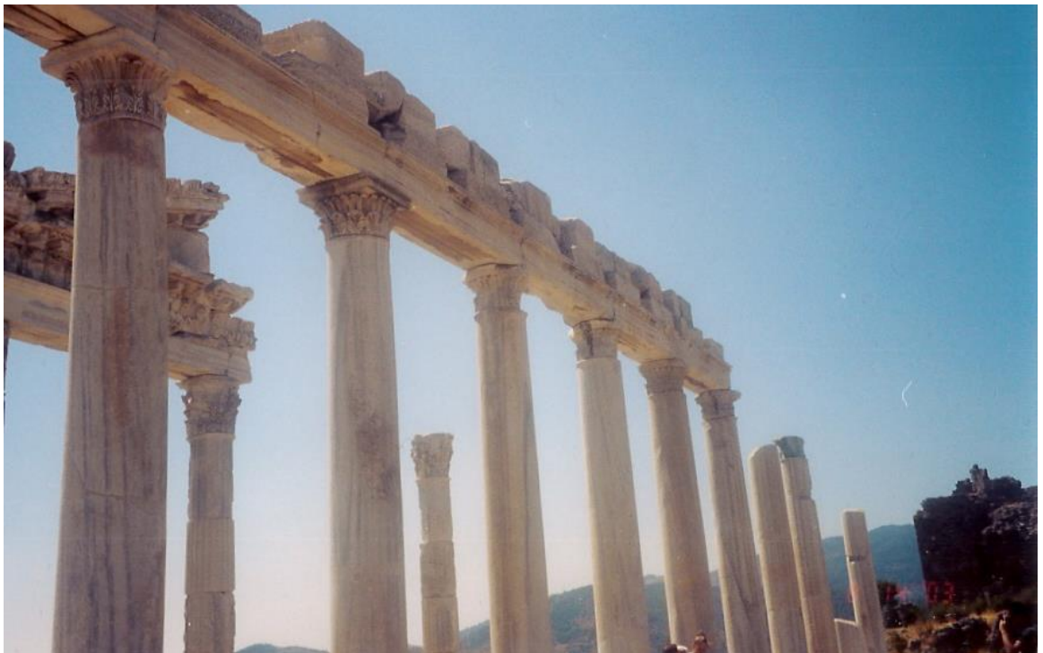
Figure 194b: the temple after the anastylosis, showing the treatment and re-assembly of fractured elements (source: Vacharopoulou -- personal photographs, 2003).
