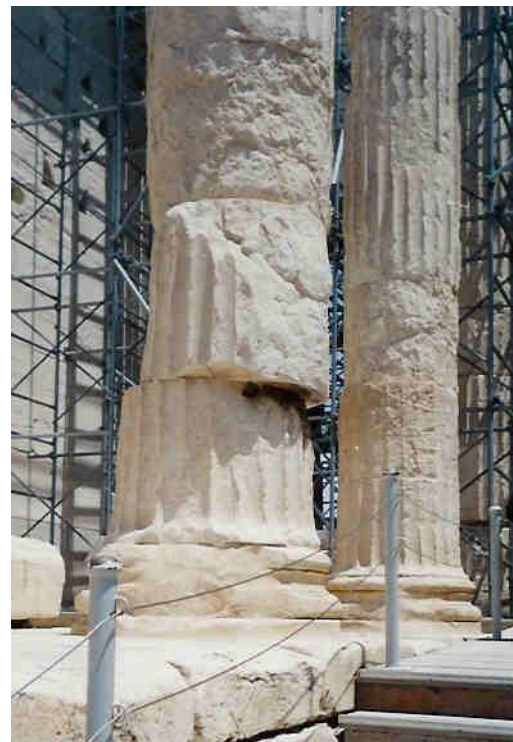
Figure 37b: example of shifted column drums (source: Vacharopoulou, personal photographs-- 2002).
