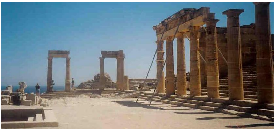
Figure 131: view of the transverse colonnade and the east corner of the restored stoa (source: Vacharopoulou -- personal photographs, 2003).
