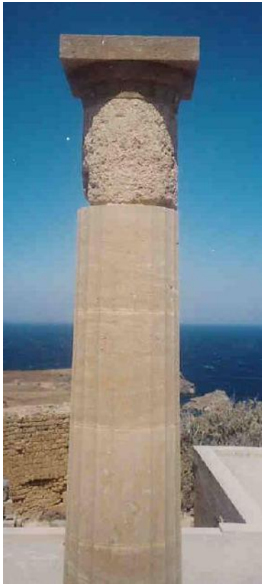
Figures 138a, b: close view of columns indicating integration of eroded drums with new ones (source: Vacharopoulou -- personal photographs, 2003).
