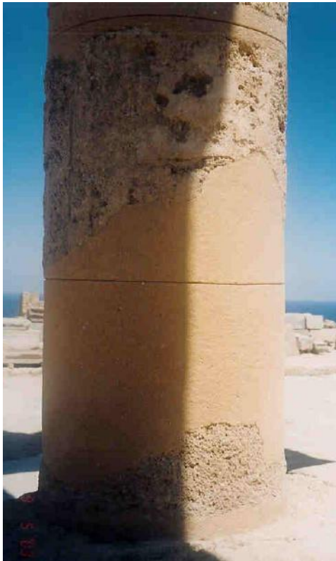
Figures 141a, b: close view of columns indicating harmonious integration, yet differentiation between original and new material (source: Vacharopoulou -- personal photographs, 2003).
