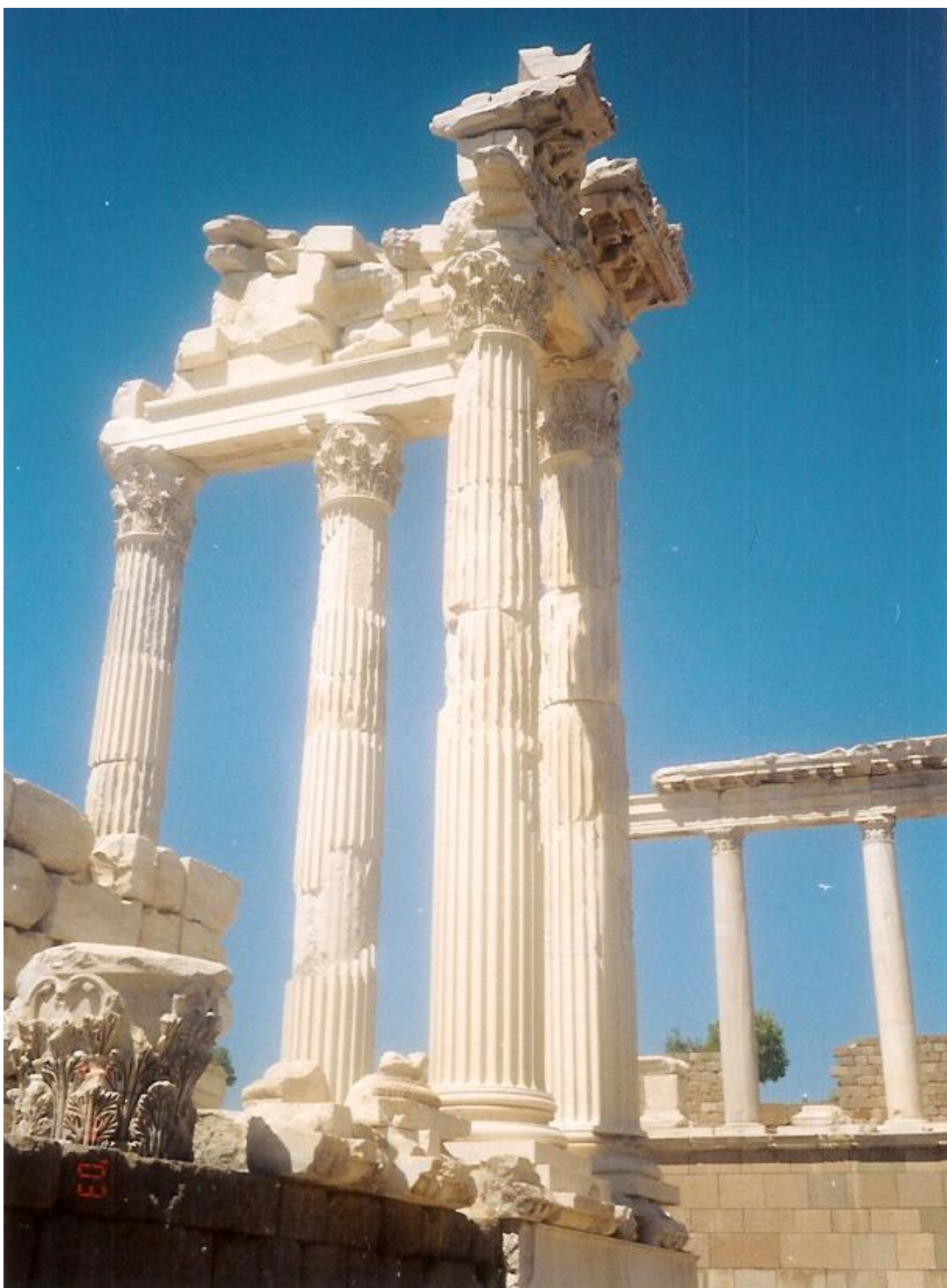
Figure 192a: anastylosis of the eastern part of the Trajaneum (source: Vacharopoulou -- personal photographs, 2003).
