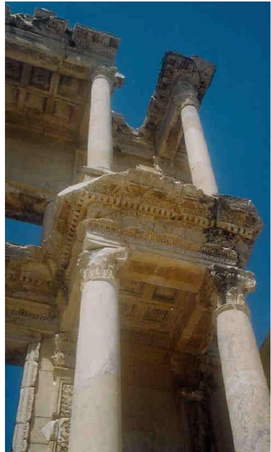
Figure 166b: restored columns of the Library, showing the colour of the new stone being suitable to the original (source: Vacharopoulou -- personal photographs, 2003)
