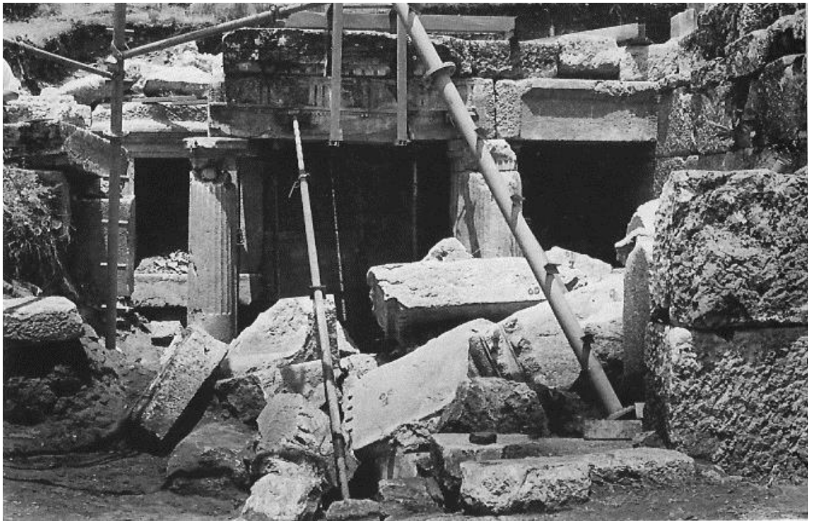
Figure 205: view of the collapsed east portico of the Nymphaeum before the anastylosis (1991) (source: Patricio and Van Balen 1993, 92).
