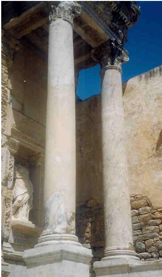
Figure 166a: restored columns of the Library, showing the colour of the new stone being suitable to the original (source: Vacharopoulou -- personal photographs, 2003).
