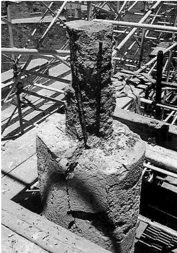
Figure 111a: nuclear of reinforced concrete revealed after the dismantling and removal of the new drum of the Italian anastylosis of 1938 (1998) (source: Pikoula 2002d, 99).
