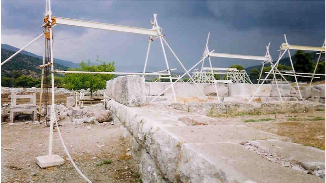
Figure 92: view of the Gymnasium Propylon showing the amount of surviving material in the building (source: Vacharopoulou -- personal photographs, 2002).
