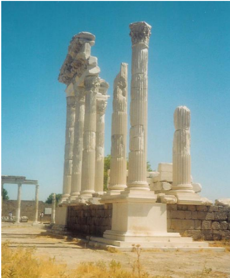
Figure 195a: View of the partial anastylosis of the Trajaneum (colonnade and entablature) (source: Vacharopoulou -- personal photographs, 2003).
