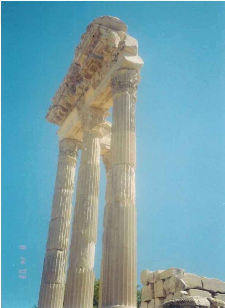
Figure 195c: View of the partial anastylosis of the Trajaneum (colonnade and entablature) (source: Vacharopoulou -- personal photographs, 2003).
