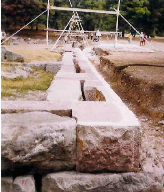
Figure 86a: anastylosis on the Gymnasium Propylon showing how exposed surfaces will be protected by reassembly of old members and integration of new ones (source: Vacharopoulou -- personal photographs, 2002).
