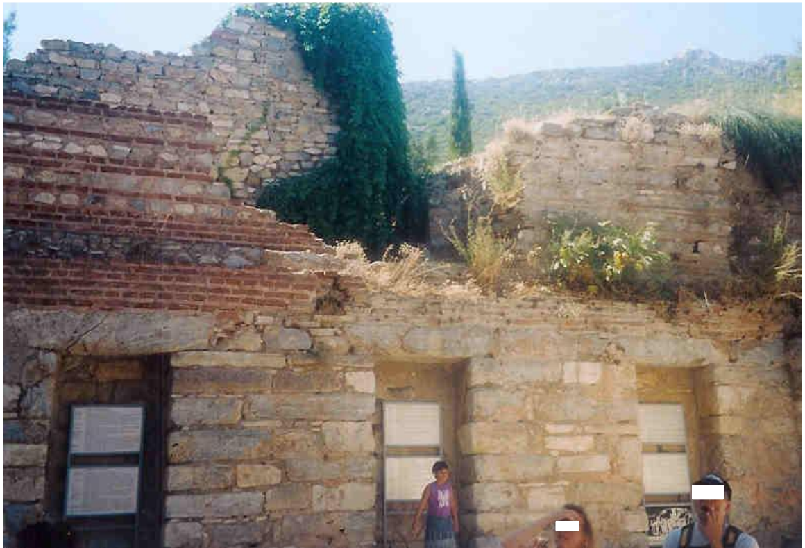
Figure 159a: The restored interior of the Library with notice boards informing about the anastylosis (source: Vacharopoulou -- personal photographs, 2003).
