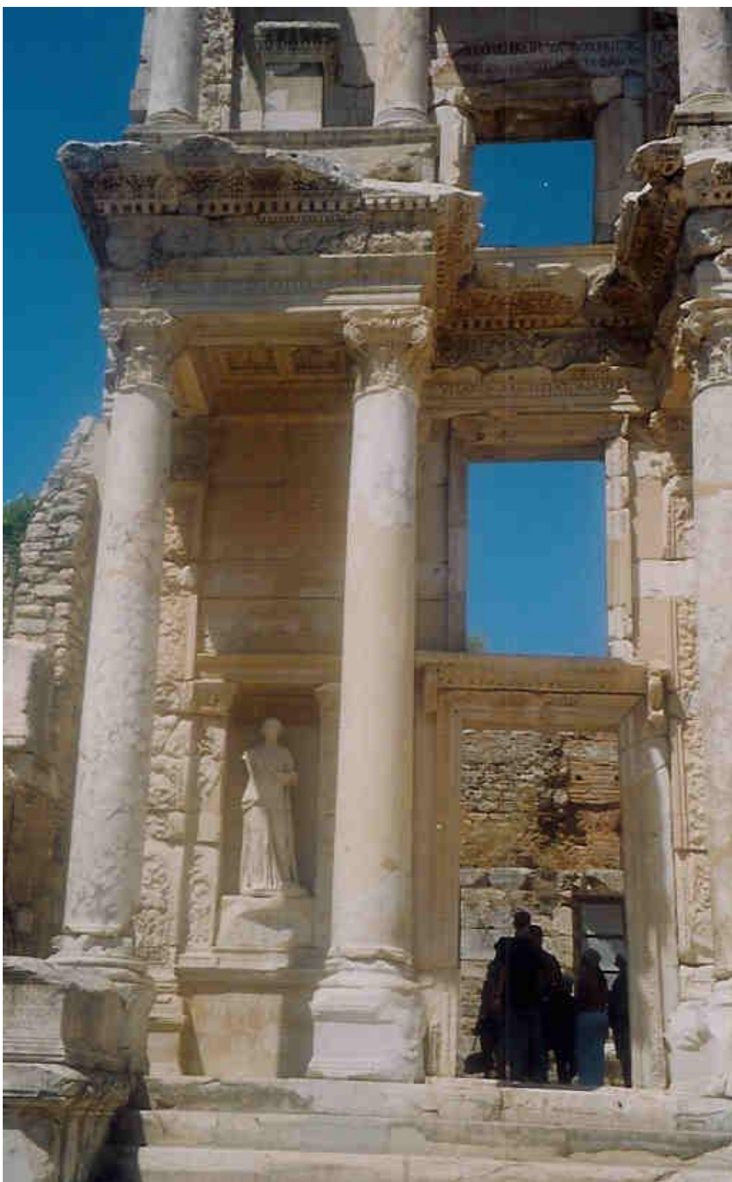
Figure 164: close view of the restored façade of the Library, showing the replacement of missing members and their differentiation from the original material (source: Vacharopoulou -- personal photographs, 2003).
