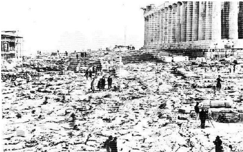
Figure 62a: the central walk before it was covered over with a thin layer of mortar (source Casanaki and Mallouchou 1985, 35).
