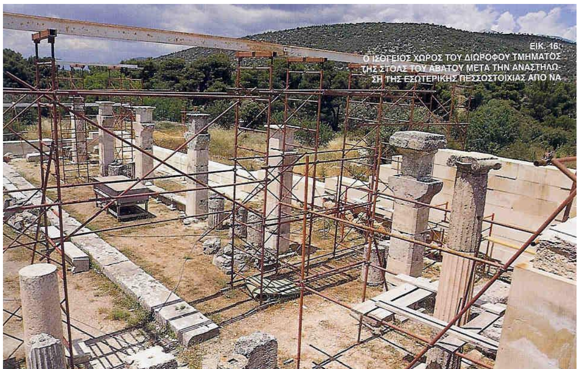
Figure 80b: the ground floor of the two-storey part of the Stoa of Avaton after anastylosis of the internal colonnade from northeast (source: Maurommatidis 1999, 33).
