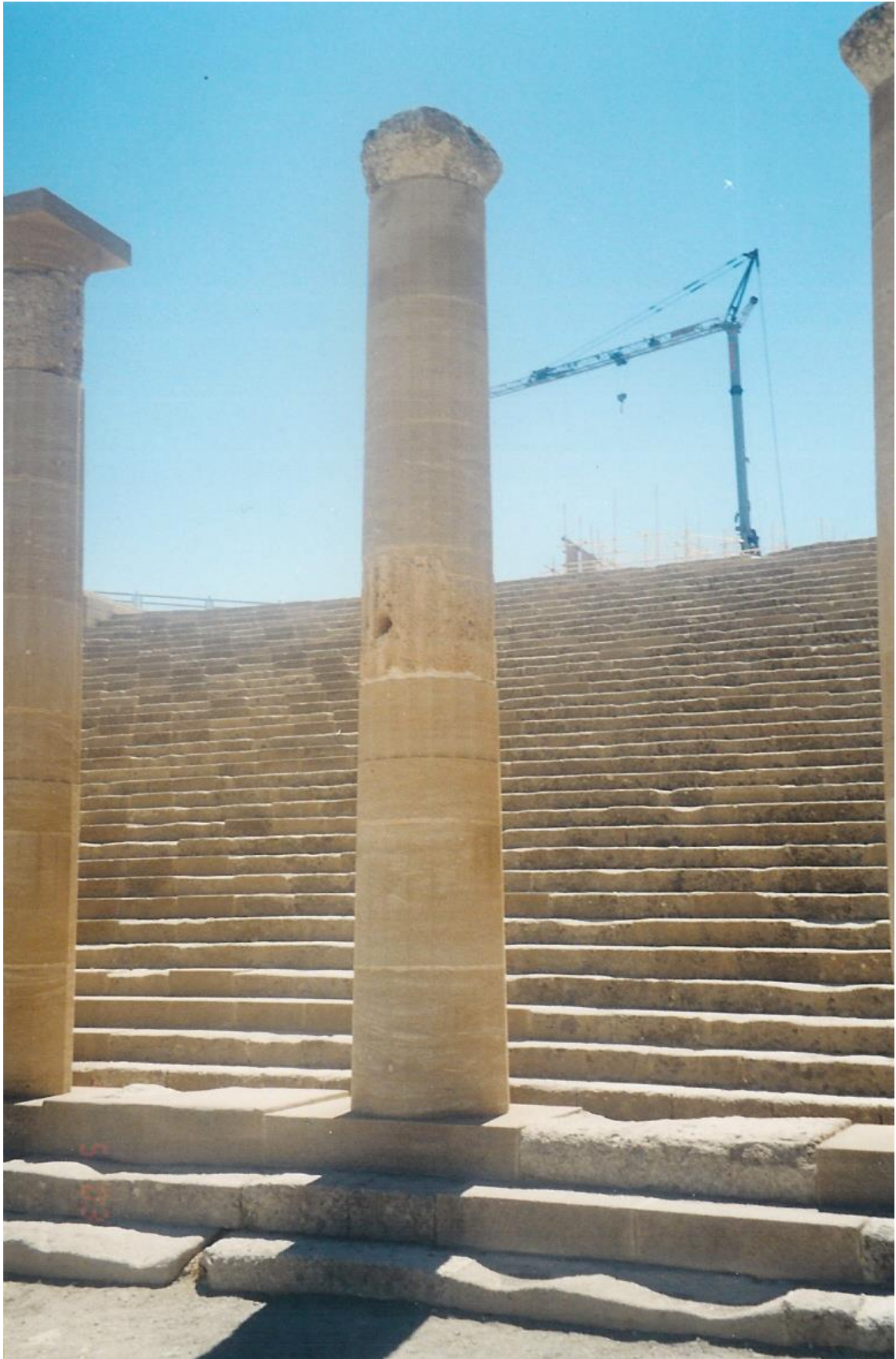
Figure 142: close view of columns indicating harmonious integration, yet differentiation between original and new material (source: Vacharopoulou -- personal photographs, 2003).
