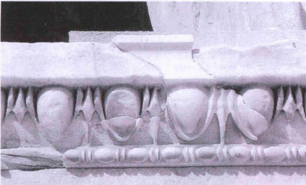
Figure 19: example of integration of new member without differentiation from the Erechtheion (source: Schmidt 1993, 245).
