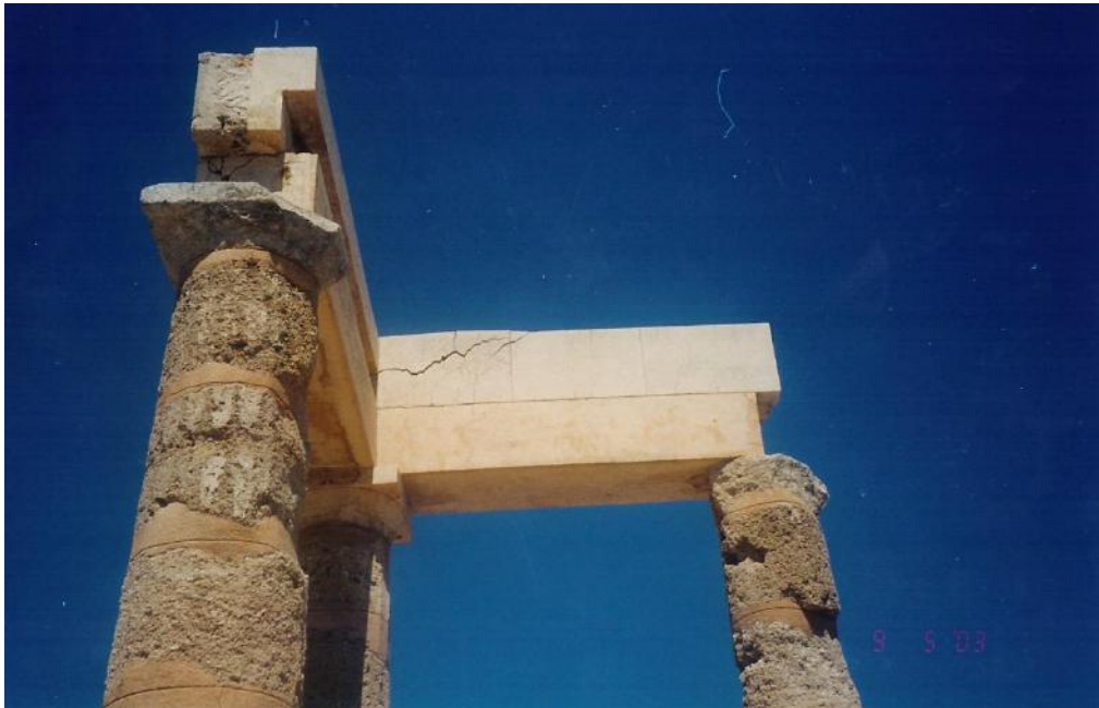
Figure 139a: close view of the entablature of the east corner of the stoa showing integration of badly preserved original material and new material (source: Vacharopoulou -- personal photographs, 2003).
