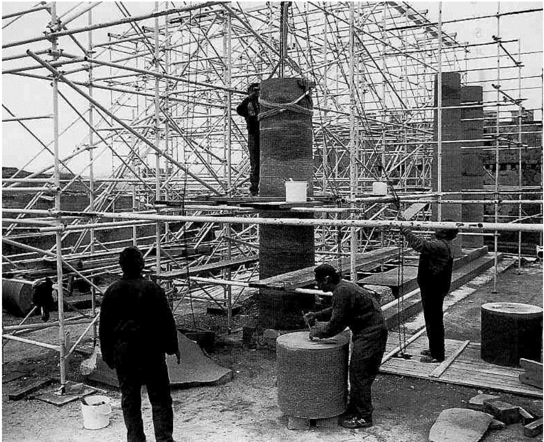
Figure 121: anastylosis of columns (1999) (source: Eleftheriou 2002a, 139).
