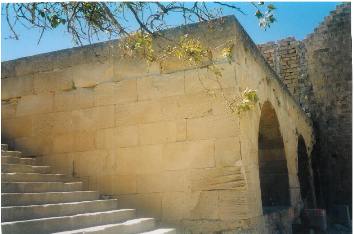
Figure 145b: View of the right vault, inside which structural members not used in the anastylosis are exhibited (source: Vacharopoulou -- personal photographs, 2003).
