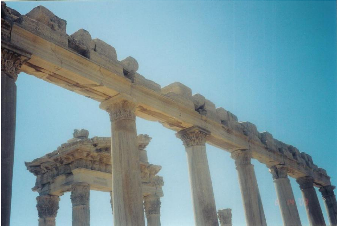
Figure 194a: the temple after the anastylosis, showing the treatment and re-assembly of fractured elements (source: Vacharopoulou -- personal photographs, 2003).
