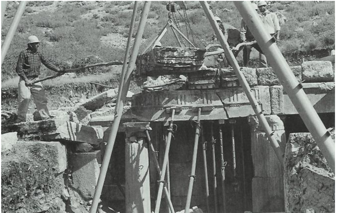
Figure 200: removal of cornice blocks (1990) (source: Waelkens 1993c, 72).
