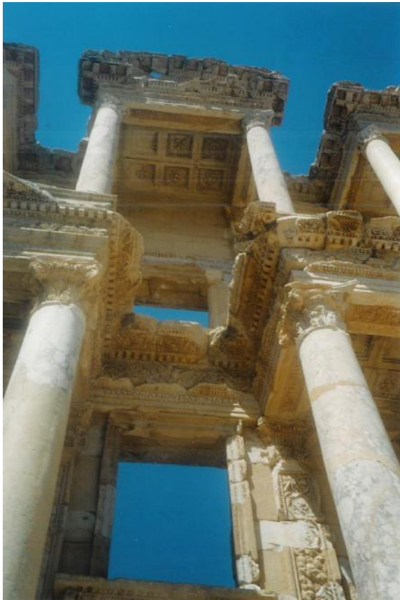
Figure 167c: close view of the restored façade of the Library showing the degree of harmonious integration and discreet differentiation between original and new members (source: Vacharopoulou -- personal photographs, 2003).
