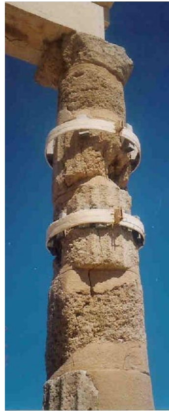
Figures 137a, b: a column of the transverse colonnade of the stoa that presents problems of structural stability (source: Vacharopoulou -- personal photographs, 2003).
