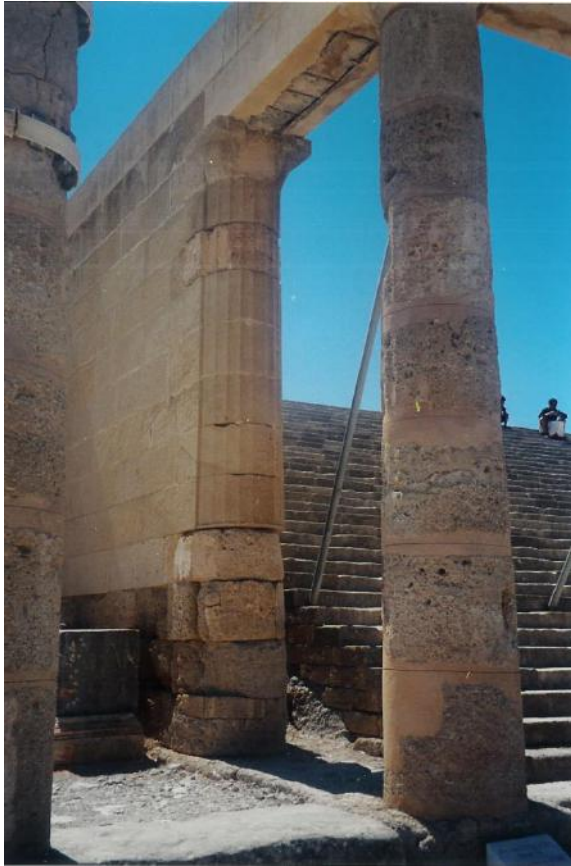
Figure 113d: view of the restored stoa and the east separating wall (source: Vacharopoulou -- personal photographs, 2003).
