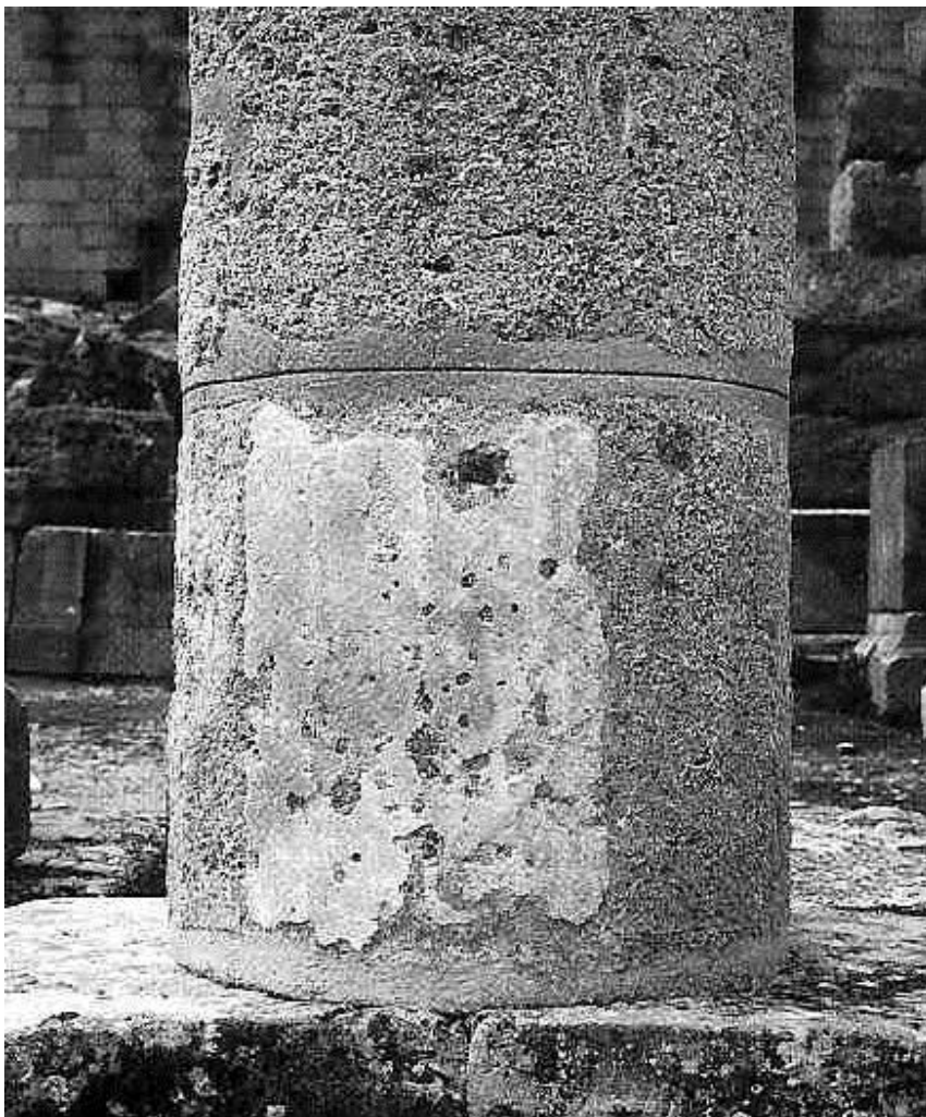
Figure 118b: detail of a column with a mortar plaster (1989) (source: Eleftheriou 2002h, 50).
