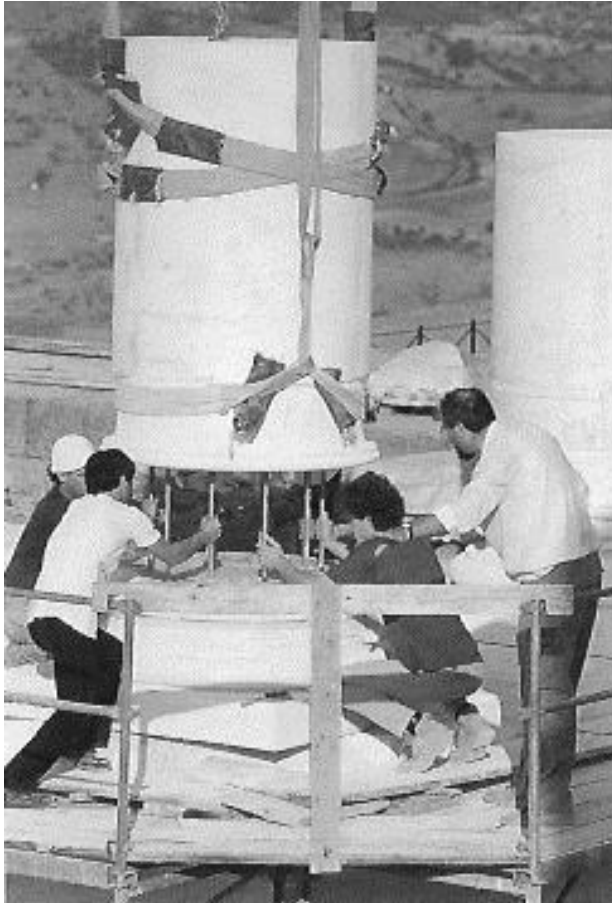
Figure 182a: joining drums and fragments of columns (source: Schmidt 1993, 175).
