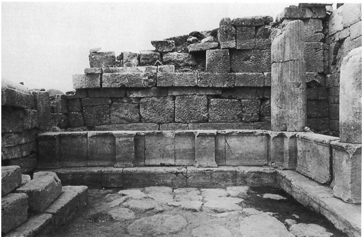
Figure 213: west portico with repaired back wall (source: Waelkens 1993c, 74).
