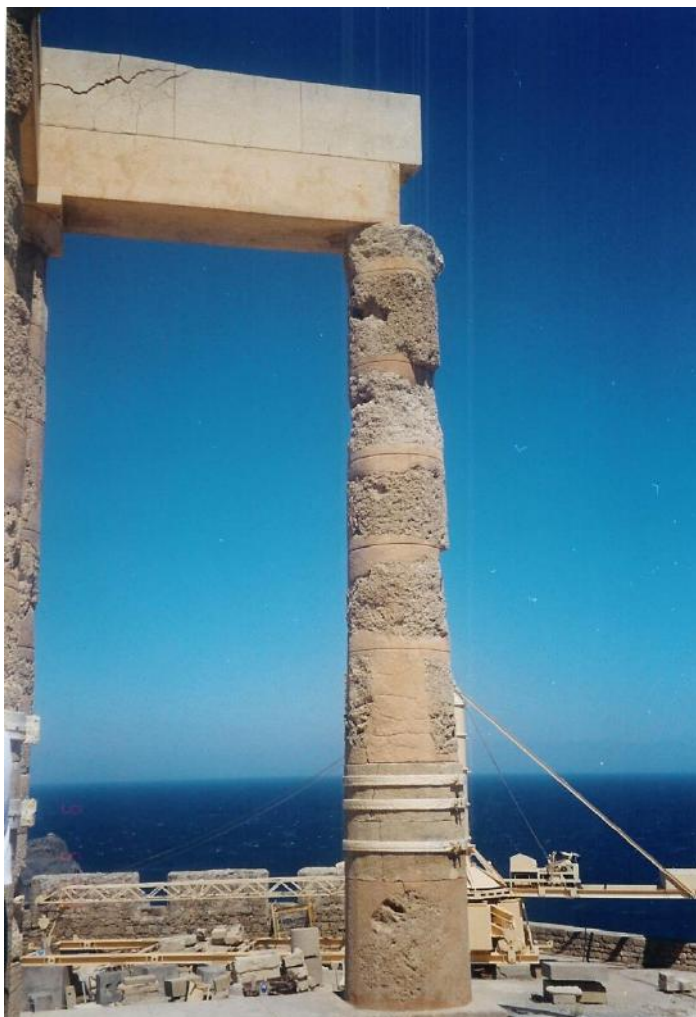
Figure 139b: close view of the entablature and a column of the east corner of the stoa showing integration of badly preserved original material and new material (source: Vacharopoulou -- personal photographs, 2003).
