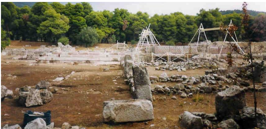
Figure 85c: anastylosis works in the Propylon of the Gymnasium
