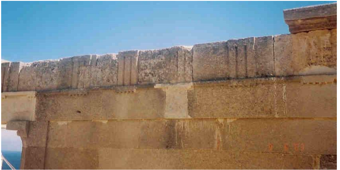
Figure 134b: close view of the restored entablature of the transverse colonnade and the east wall of the stoa, showing the integration of new and original material (source: Vacharopoulou -- personal photographs, 2003).
