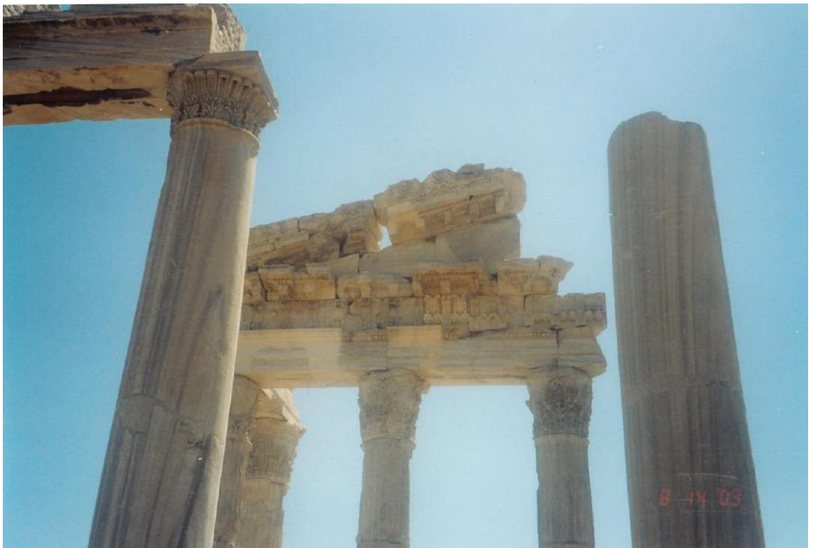
Figure 191b: example of the fragmentary anastylosis, only where the preserved material allowed it (source: Vacharopoulou -- personal photographs, 2003).
