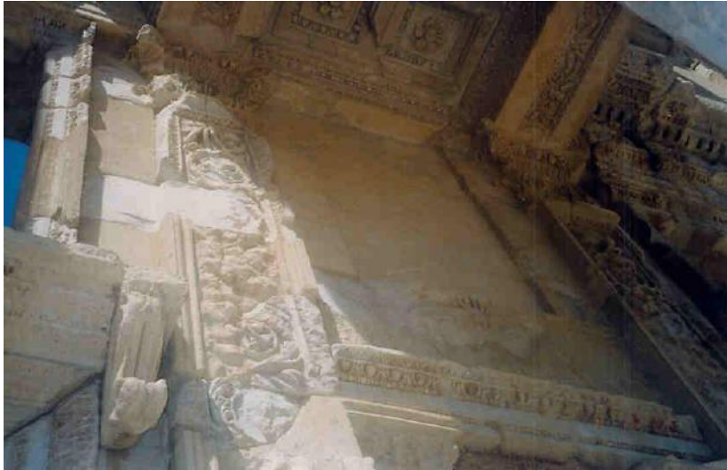
Figure 168a: close view of restored parts of the Library's façade, showing the degree to which ornamentation was copied (source: Vacharopoulou -- personal photographs, 2003).
