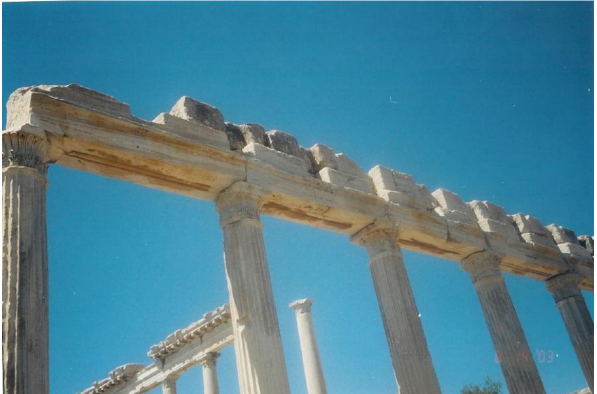
Figure 193a: close view of the restored entablature of the eastern part of the Trajaneum (source: Vacharopoulou -- personal photographs, 2003).
