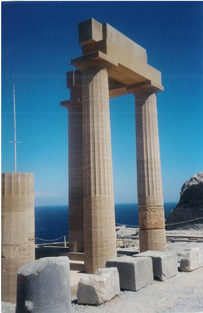
Figure 133a: close view of the east corner of the restored stoa (source: Vacharopoulou -- personal photographs, 2003).
