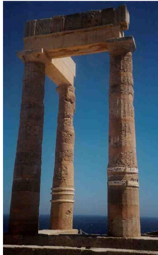
Figure 132b: view of the east corner of the restored stoa (source: Vacharopoulou -- personal photographs, 2003).
