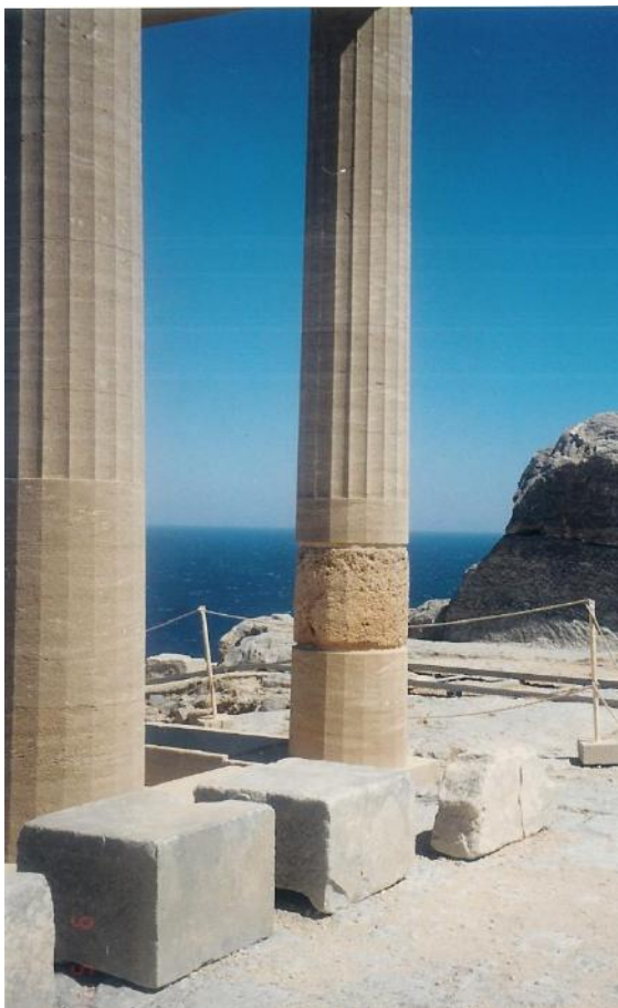
Figure 138c: close view of columns indicating integration of eroded drums with new ones (source: Vacharopoulou -- personal photographs, 2003).
