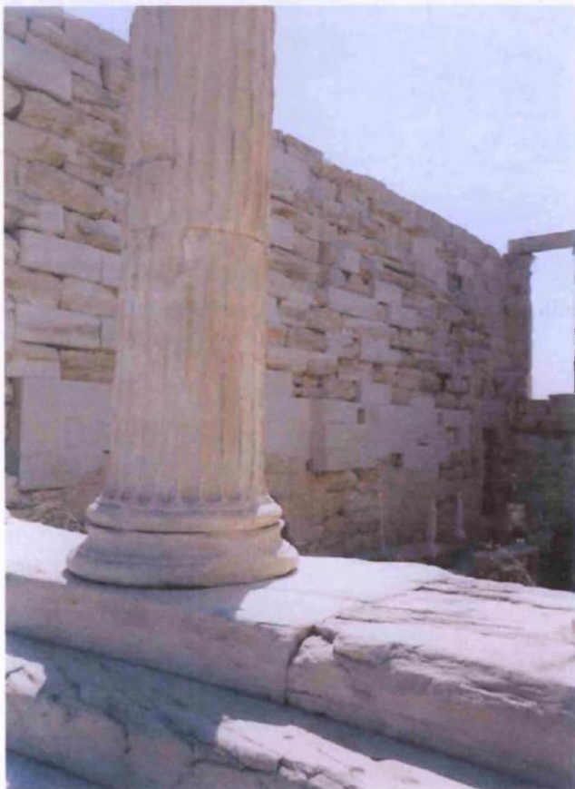
Figure 24: view of the interior of the restored Erechtheion, showing the use of Pentelic marble for additions and missing members (source: Vacharopoulou, personal photographs -- 2002).
