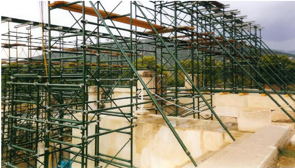
Figure 81a: anastylosis works in the Avaton Stoa with integration of new and original members (source: Vacharopoulou -- personal photographs, 2002).
