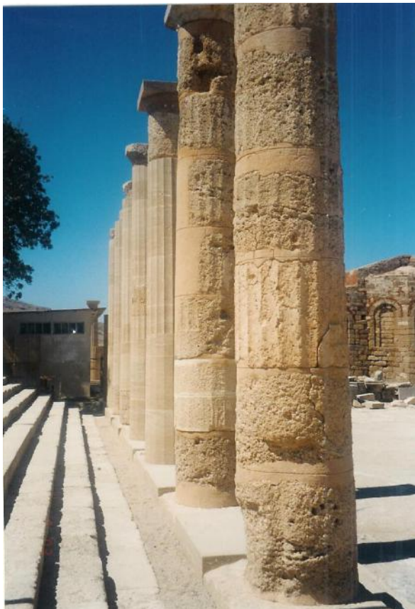
Figure 114: close view of the restored colonnade (source: Vacharopoulou -- personal photographs, 2003).
