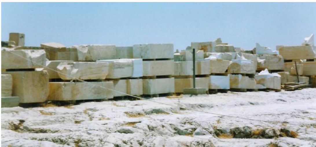
Figure 46c: architectural members, original and new, prepared for their integration into the Parthenon (2003) (source: Vacharopoulou -- personal photographs, 2003).
