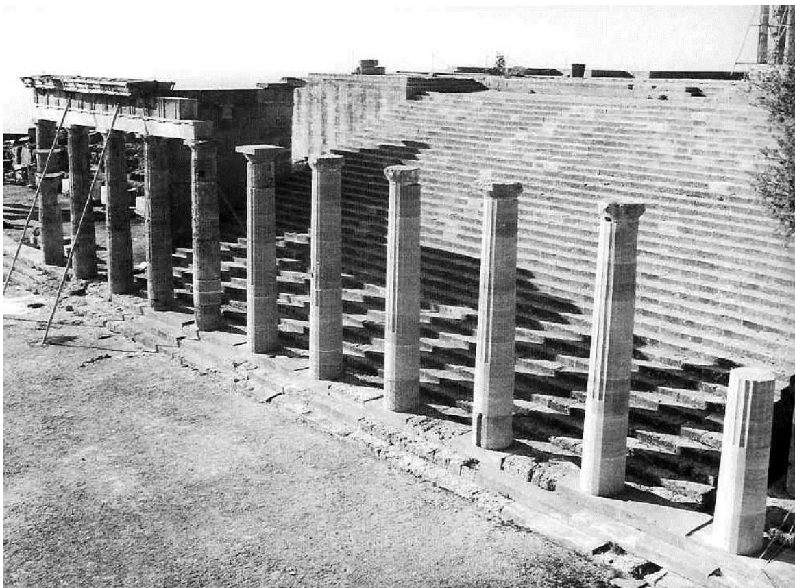
Figure 106b: the free part of the transverse colonnade after the intervention (1997) (source: Eleftheriou 2002a, 116).
