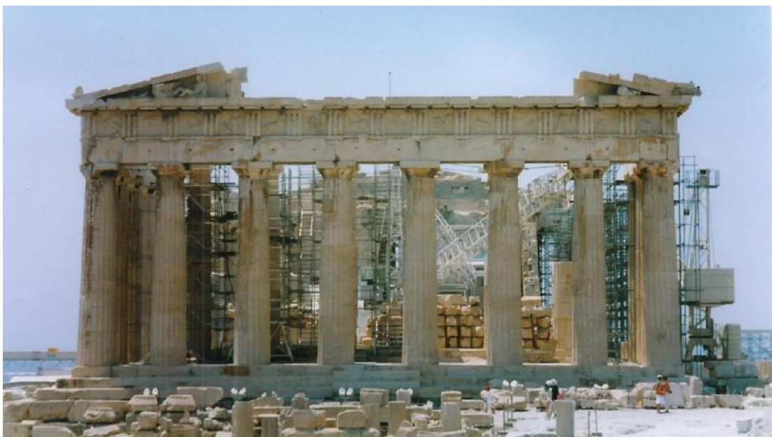
Figure 53d: the east side of the Parthenon during anastylosis (source: Vacharopoulou -- personal photographs, 2002).
