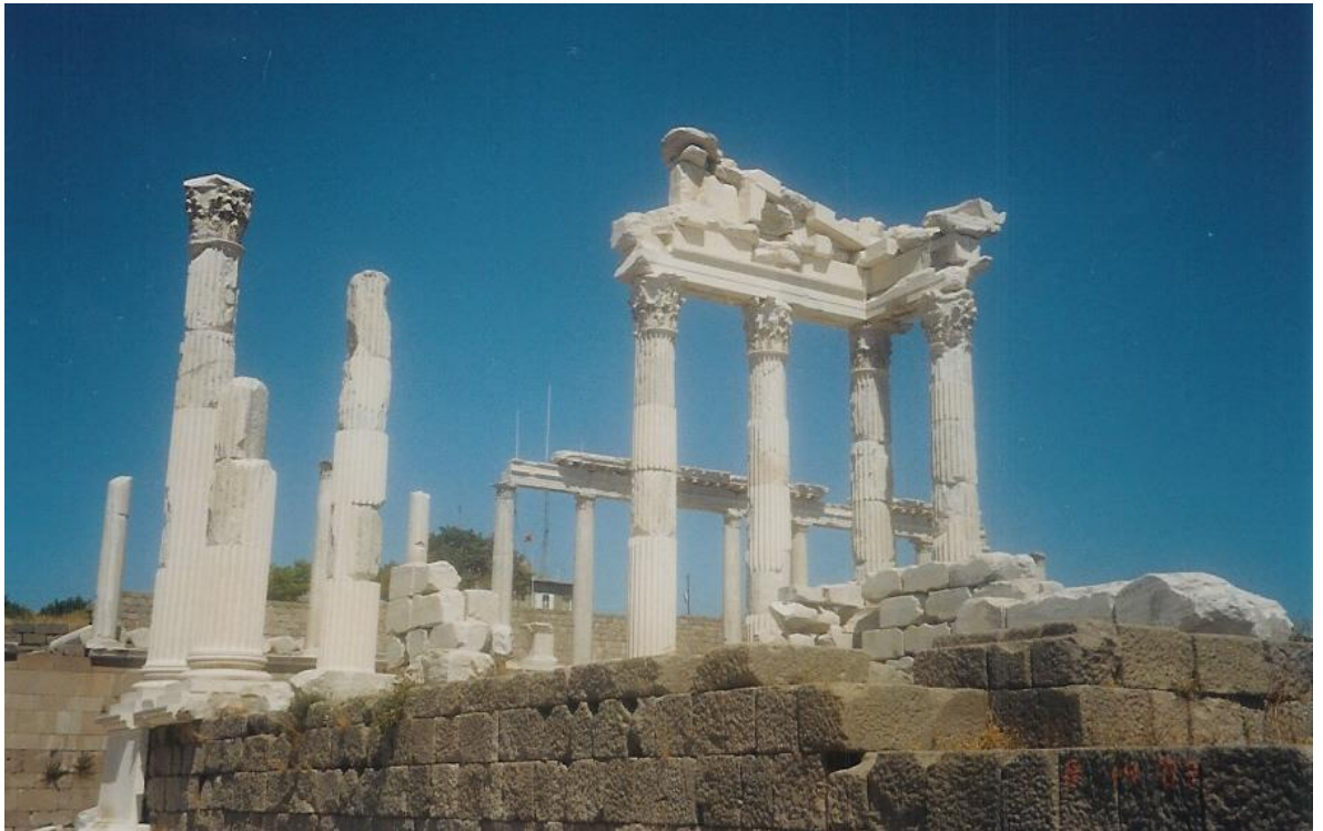
Figure 191a: example of the fragmentary anastylosis, only where the preserved material allowed it (source: Vacharopoulou -- personal photographs, 2003).
