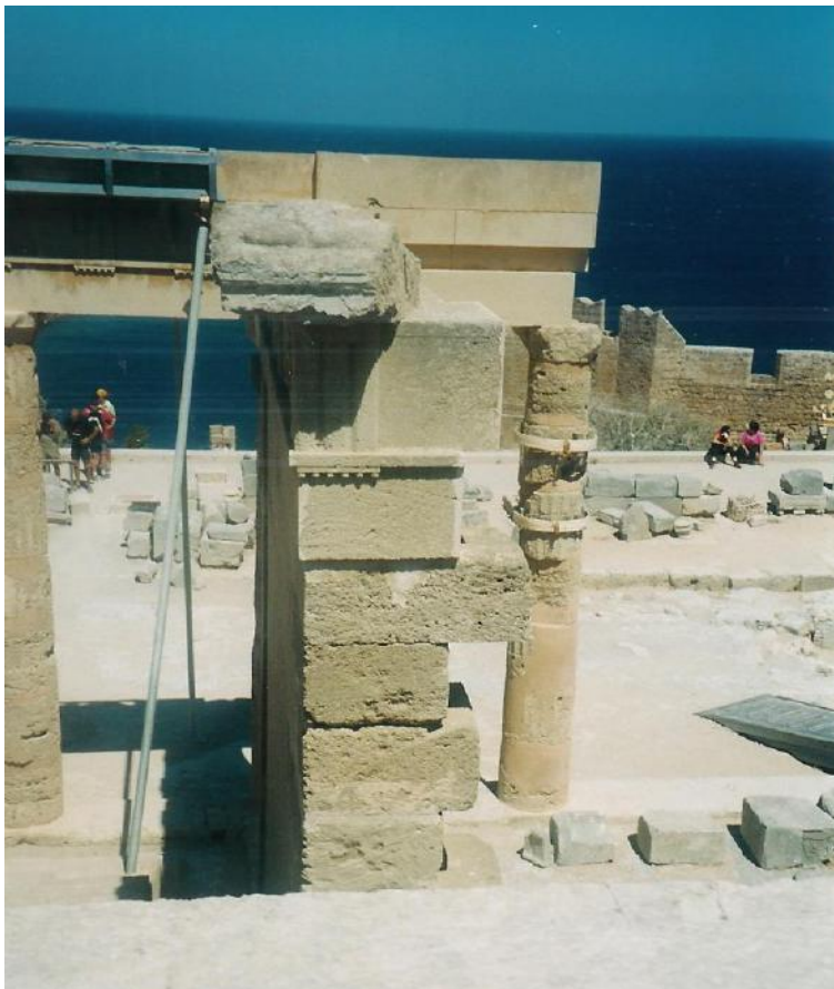
Figure 128b: close view of the east side of the restored transverse colonnade and part of the restored east wall of the Stoa (source: Vacharopoulou -- personal photographs, 2003).
