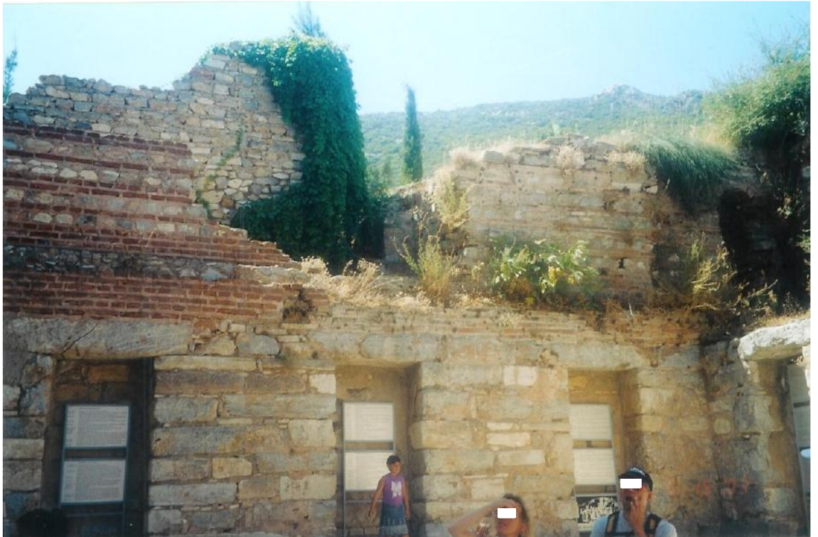
Figure 170a: the interior of the restored Library with notice boards providing information on the monument (source: Vacharopoulou -- personal photographs, 2003).
