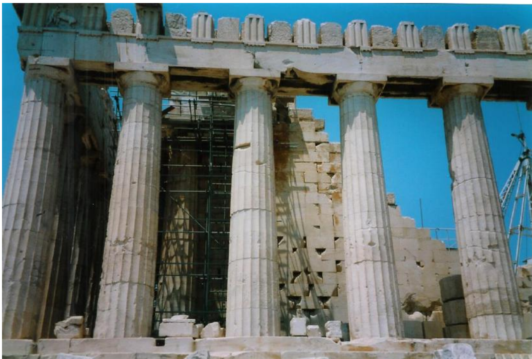
Figure56c: close view of the south side of the Parthenon during anastylosis (source: Vacharopoulou -- personal photographs, 2002).
