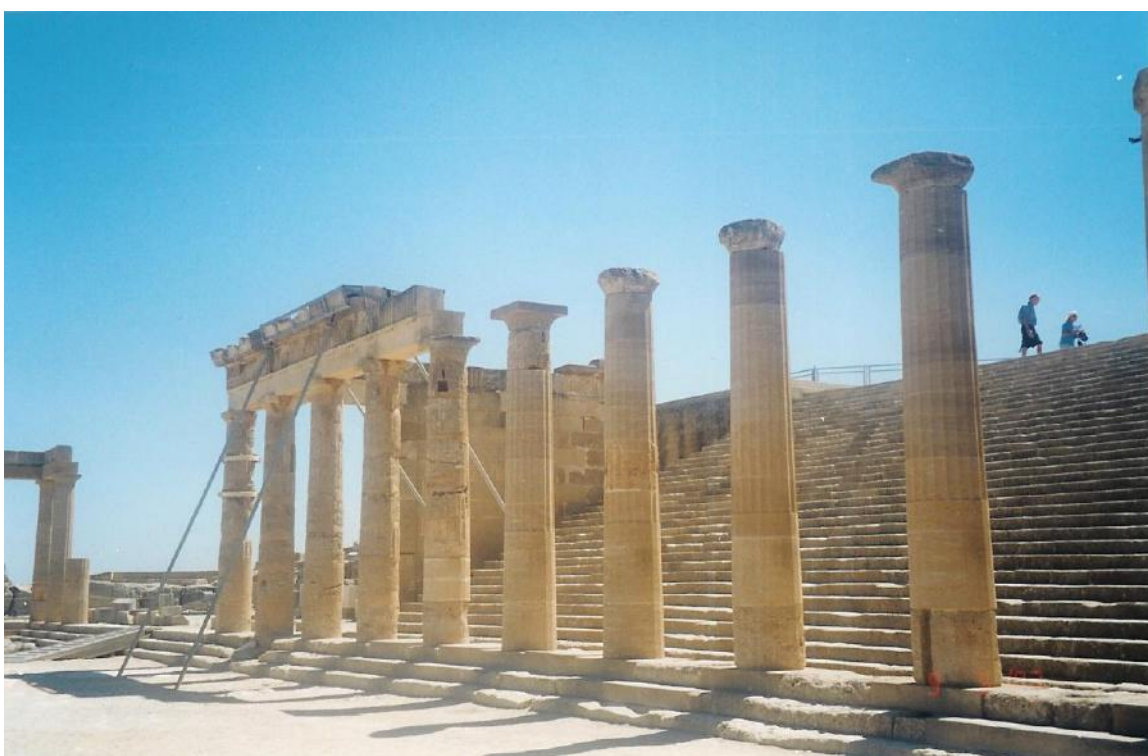
Figure 112b: view of the restored transverse colonnade of the stoa (source: Vacharopoulou -- personal photographs, 2003).
