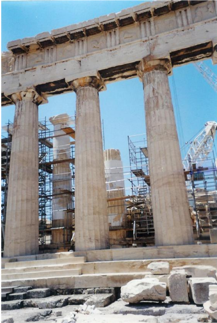
Figure 53c: close view of the east side of the Parthenon during anastylosis (source: Vacharopoulou -- personal photographs, 2002).
