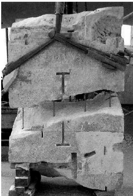
Figure 43: joining two parts using titanium rods for reinforcement (source: Maurommatis 2003, 31).
