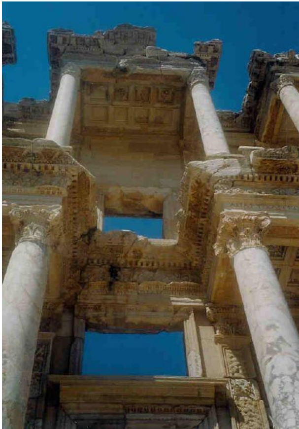
Figure 167b: close view of the restored façade of the Library showing the degree of harmonious integration and discreet differentiation between original and new members (source: Vacharopoulou -- personal photographs, 2003).
