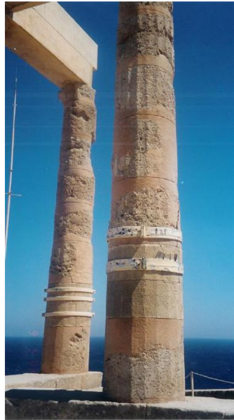
Figures 136a, b: the east corner of the stoa that presents problems of structural stability (source: Vacharopoulou -- personal photographs, 2003).
