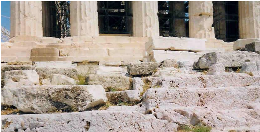
Figure 66a: detail of the stylobate and the crepis of the south side of the Parthenon (source: Vacharopoulou -- personal photographs, 2002).
