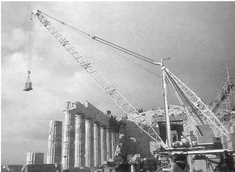
Figure 50: the derrick crane in the interior of the Parthenon (photo by Zambas, 1985) (source: SRAM 2002, 6).
