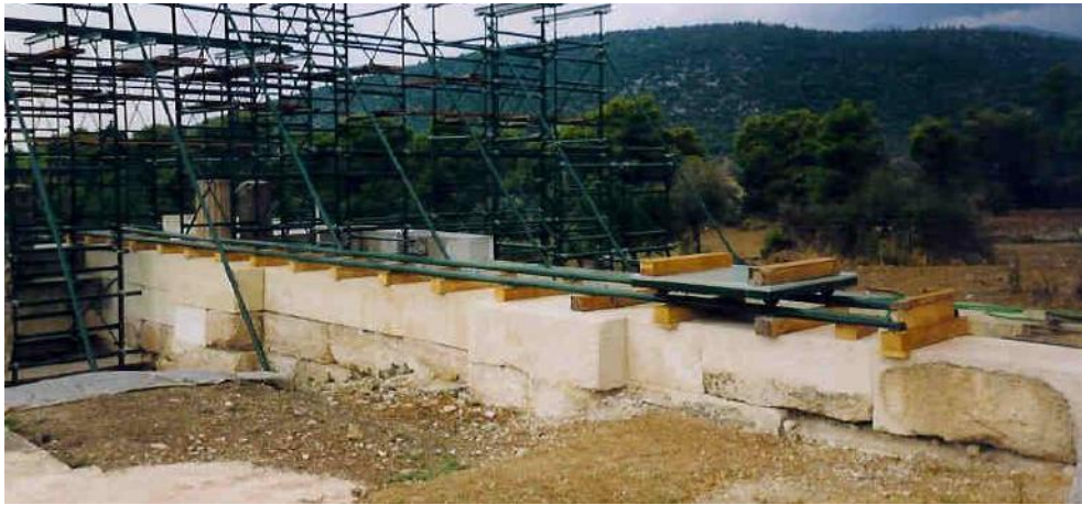
Figure 77a: anastylosis works in the Avaton Stoa, showing re-integrations and additions of stone members (source: Vacharopoulou -- personal photographs, 2002).
