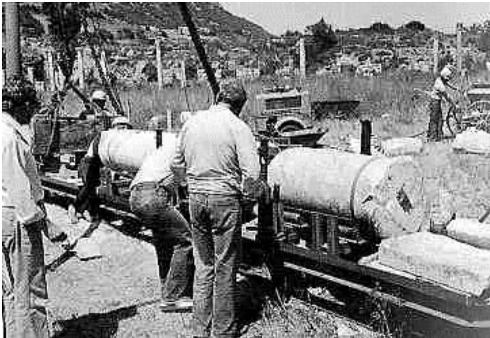
Figure 161b: working on new and old members to connect them (source: Schmidt 1993, 286).
