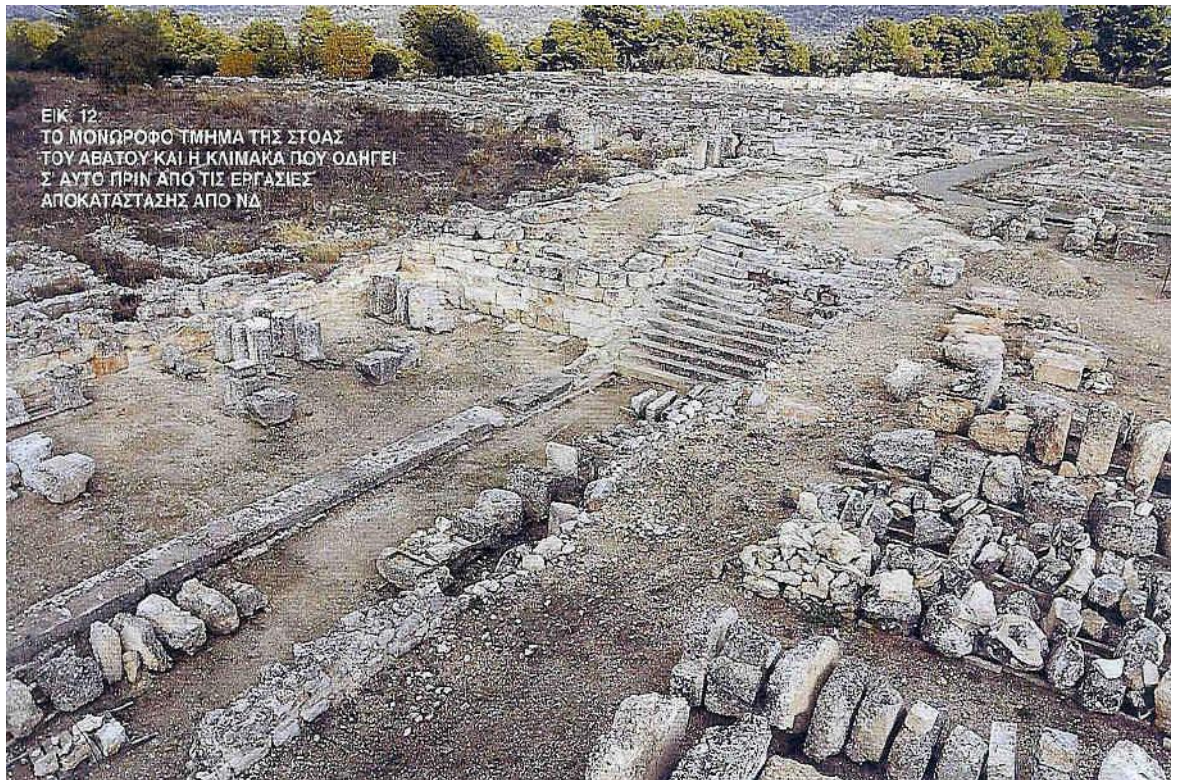
Figure 79a: the one-story part of the Stoa of Avaton and the staircase that leads to it before the works of restoration from the northwest (source: Maurommatidis 1999, 29).
