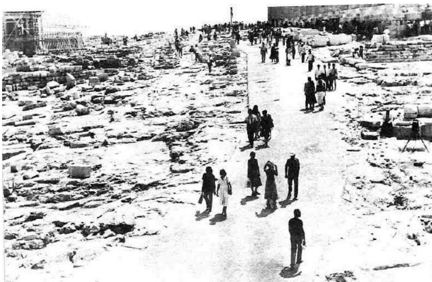
Figure 62b: the central walk after it was covered over with a thin layer of mortar (1981) (source Casanaki and Mallouchou 1985, 35).
