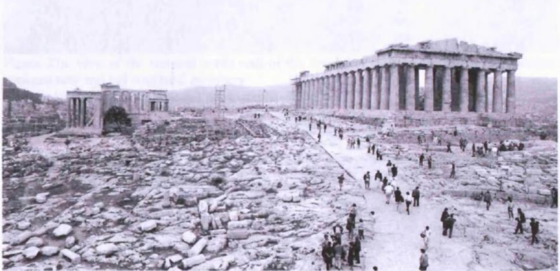
Figure 25b: general view of the Acropolis path, after it was covered with a thin layer of mortar (1987) (source: Maurommatis 2003, 15).
