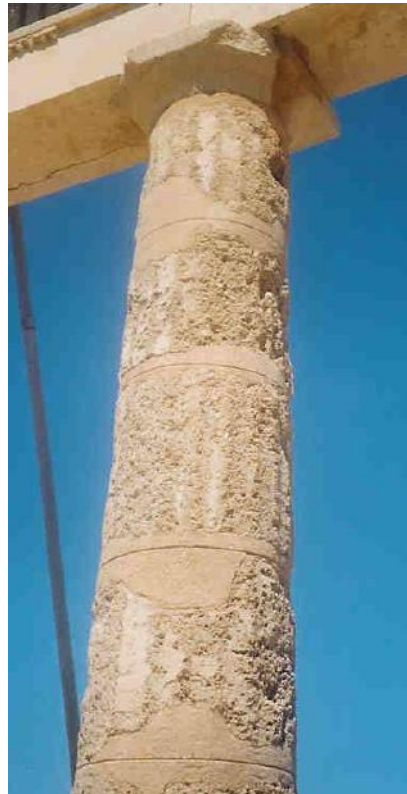
Figures 141a, b: close view of columns indicating harmonious integration, yet differentiation between original and new material (source: Vacharopoulou -- personal photographs, 2003).
