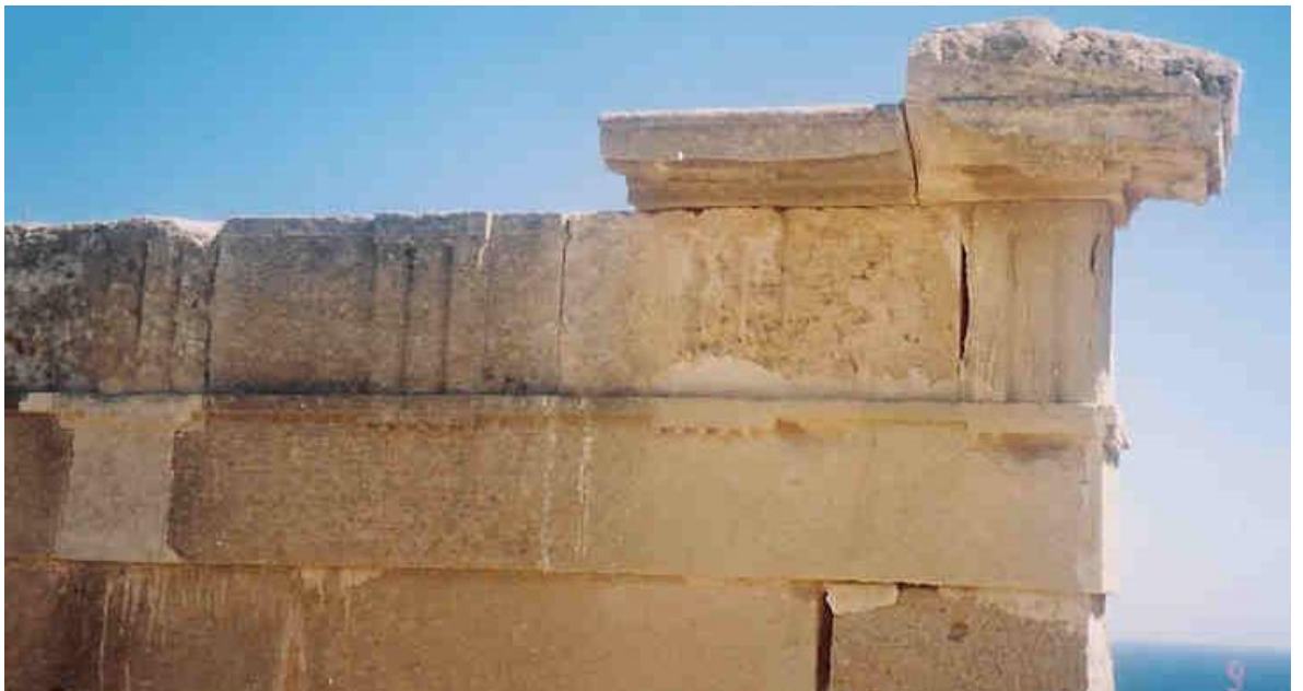
Figure 134c: close view of the restored entablature of the transverse colonnade and the east wall of the stoa, showing the integration of new and original material (source: Vacharopoulou -- personal photographs, 2003).
