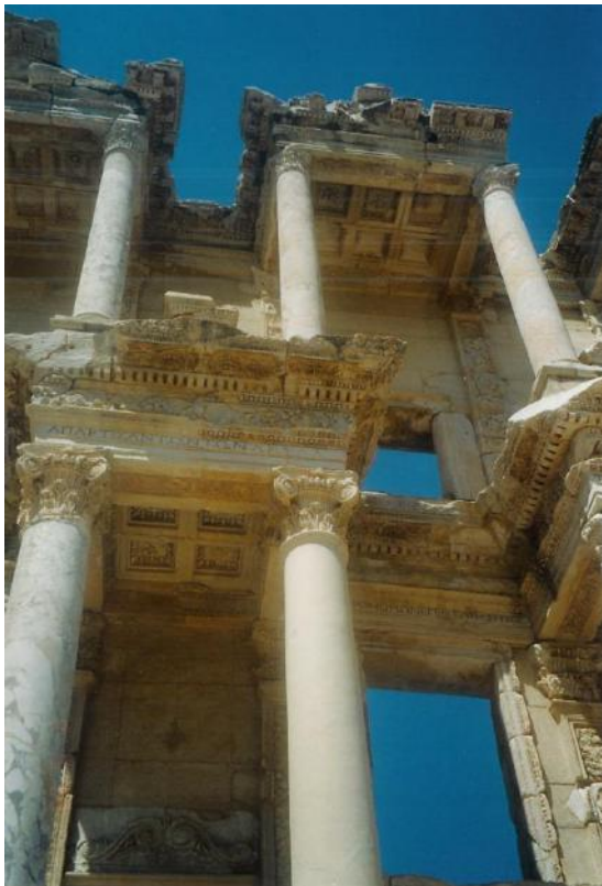
Figure 167d: close view of the restored façade of the Library showing the degree of harmonious integration and discreet differentiation between original and new members (source: Vacharopoulou -- personal photographs, 2003).
