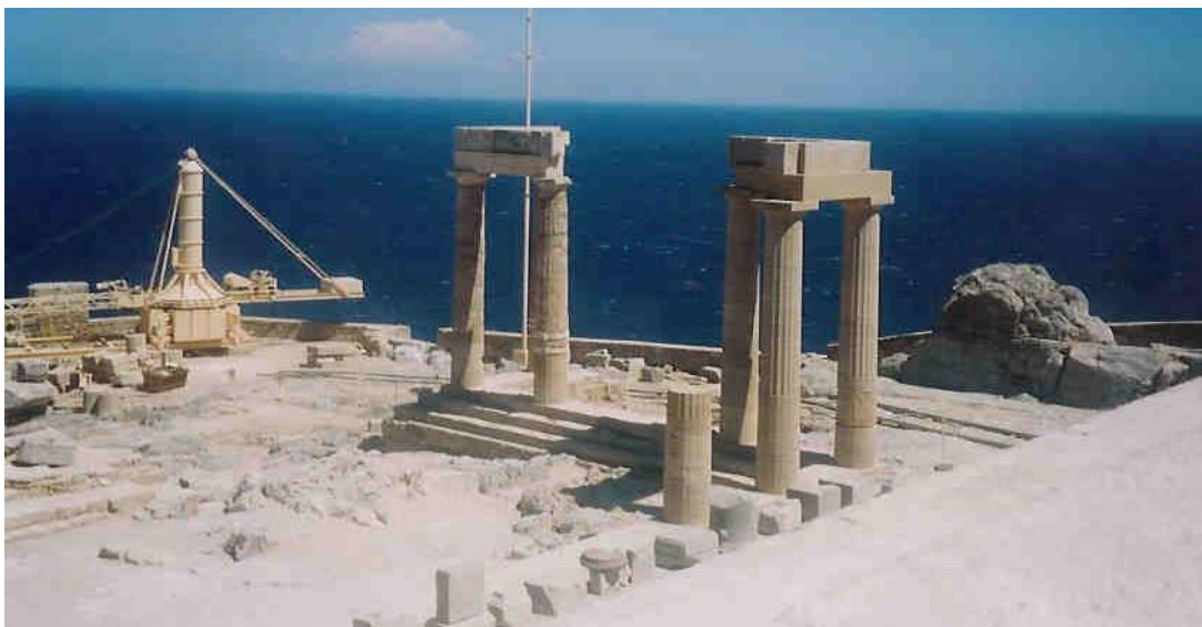
Figure 130: view of the east corner of the restored stoa (source: Vacharopoulou -- personal photographs, 2003).
