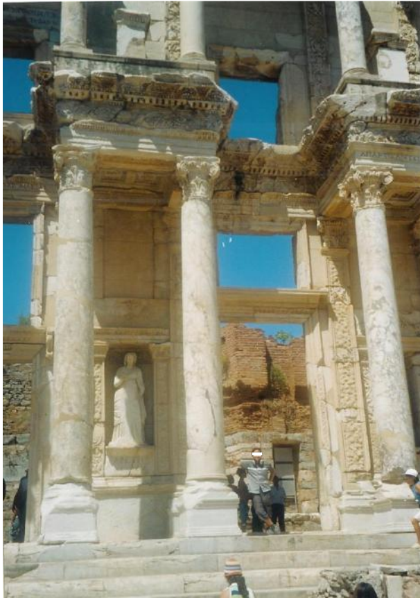
Figure 165a: close view of the restored façade of the Library, showing the replacement of missing members and their differentiation from the original material (source: Vacharopoulou -- personal photographs, 2003).
