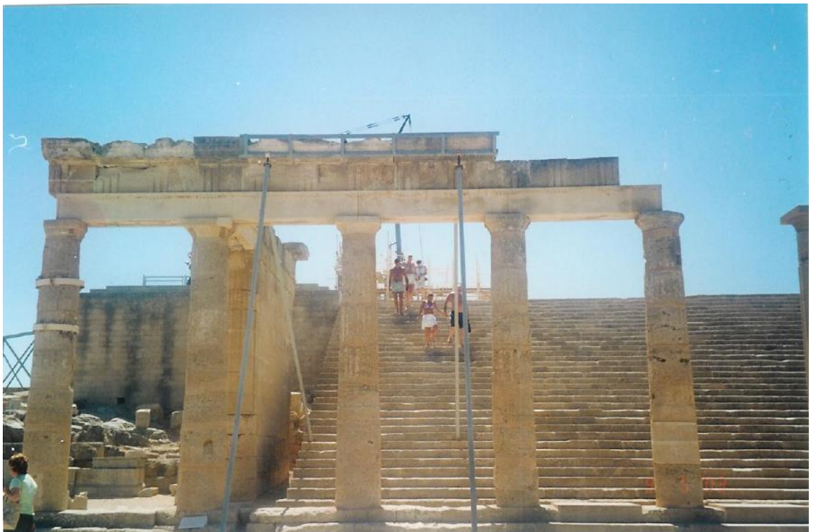
Figure 113a: view of the restored stoa and the east separating wall (source: Vacharopoulou -- personal photographs, 2003).
