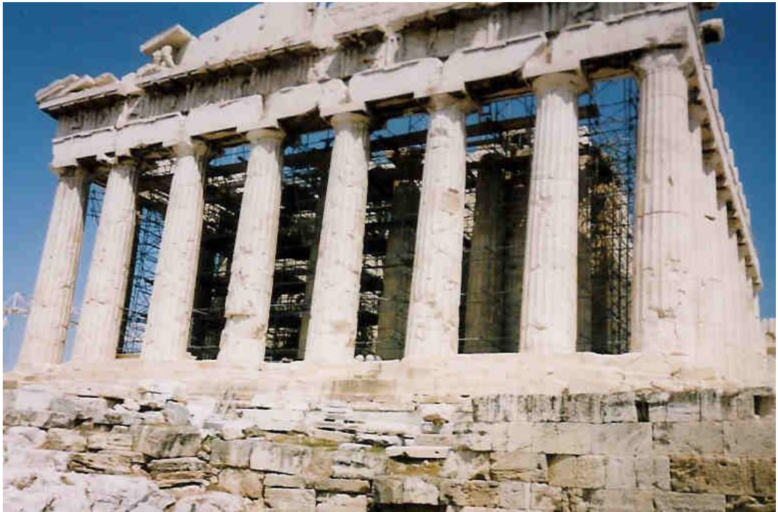
Figure 54a: the west side of the Parthenon during anastylosis (source: Vacharopoulou -- personal photographs, 2002).
