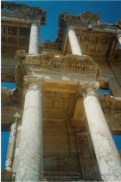
Figure 167a: close view of the restored façade of the Library showing the degree of harmonious integration and discreet differentiation between original and new members (source: Vacharopoulou -- personal photographs, 2003).
