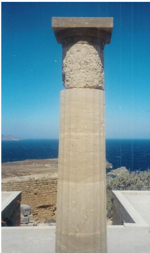
Figure 141e: close view of a column indicating harmonious integration, yet differentiation between original and new material (source: Vacharopoulou -- personal photographs, 2003).
