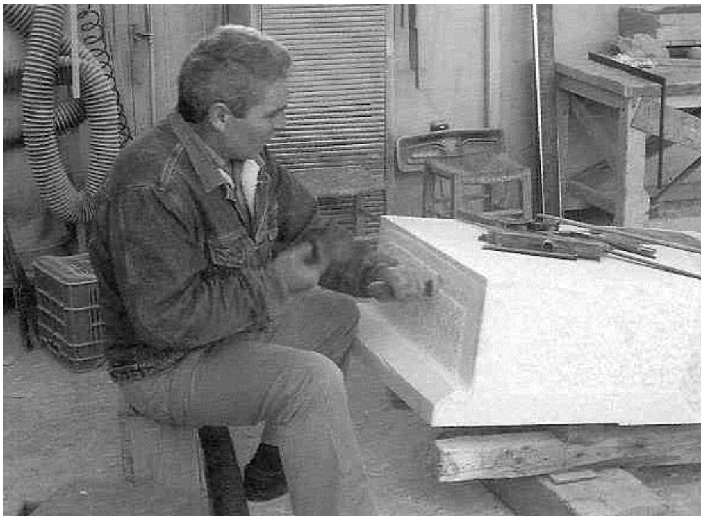
Figure 40: carving a new marble filling in a 'thranos' of the Parthenon opisthodomos (photo by Koufopoulos, 1993) (source: SRAM 2002, 22).
