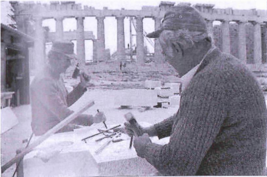
Figure 18: cutting supplementary architectural members for the Erechtheion (1985) (source: Maurommatis 2003, 31).
