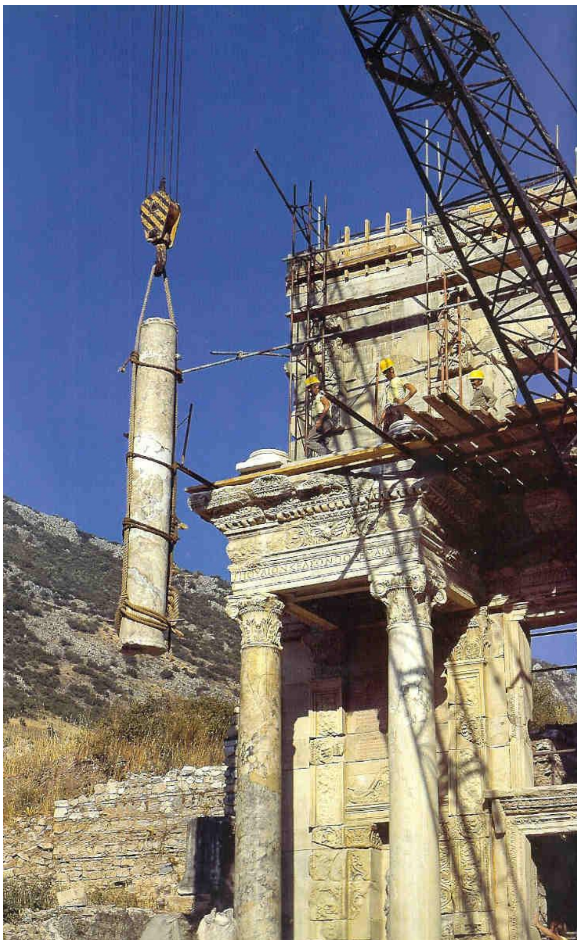
Figure 163: re-assembly of members during the anastylosis (source: Hueber 1997, 2).
