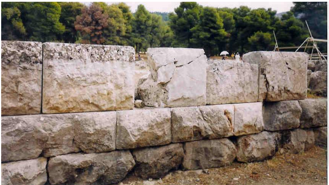
Figure 93: view of restored stone members of the Propylon of the Gymnasium (source: Vacharopoulou -- personal photographs, 2002).
