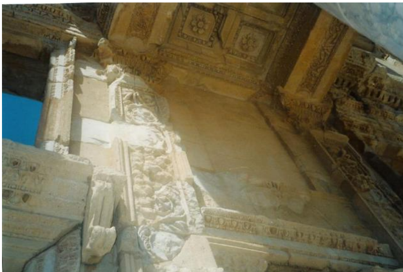
Figure 168c: close view of restored parts of the Library's façade, showing the degree to which ornamentation was copied (source: Vacharopoulou -- personal photographs, 2003).
