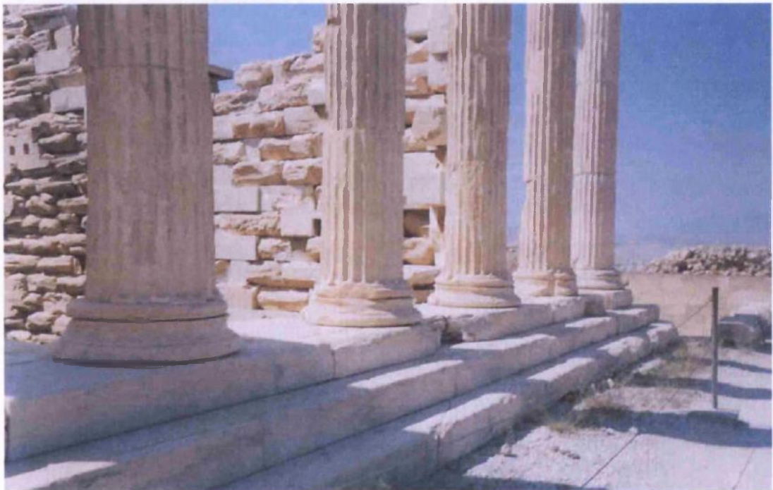
Figure 27b: view of the restored interior of the Erechtheion, showing the contrast between the shattered older members and the incorporated new ones (source: Vacharopoulou, personal photographs -- 2002).
