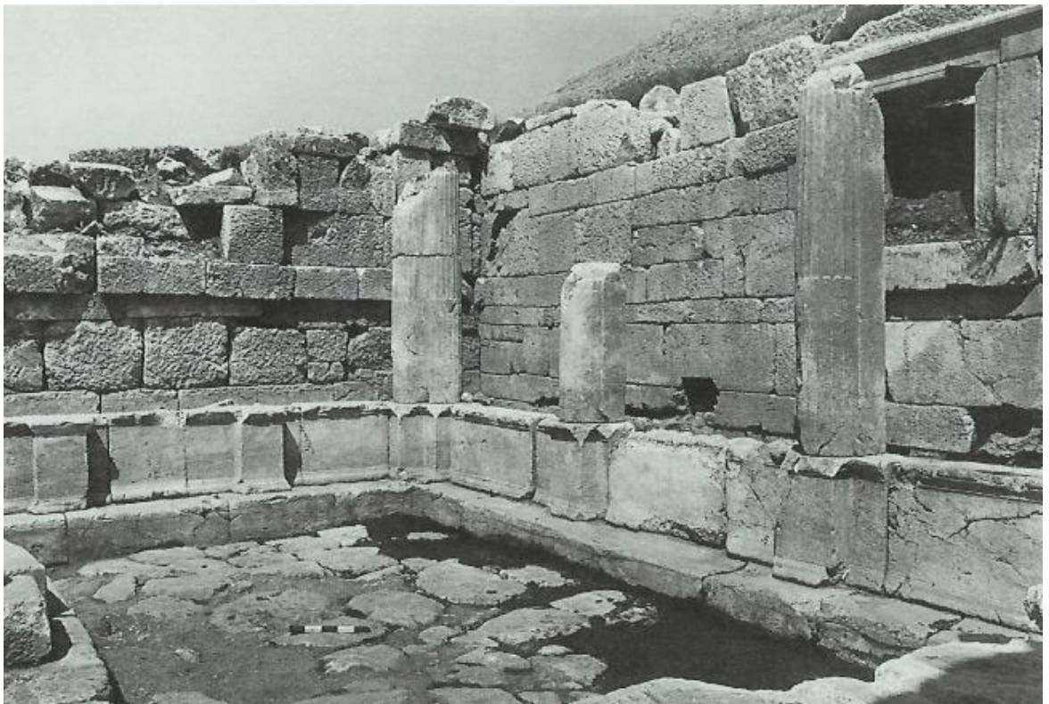
Figure 203: drawing basin of the fountain: west (left) and north portico (right) (before anastylosis) (source: Waelkens 1993c, 64).
