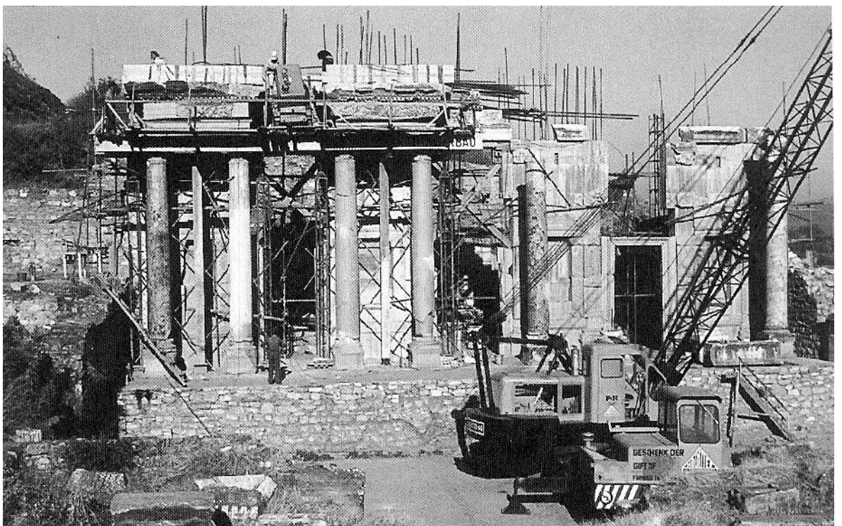
Figure 155: erection of the south ground floor architrave (1975) (source: Wiplinger and Wlach 1996, 124).
