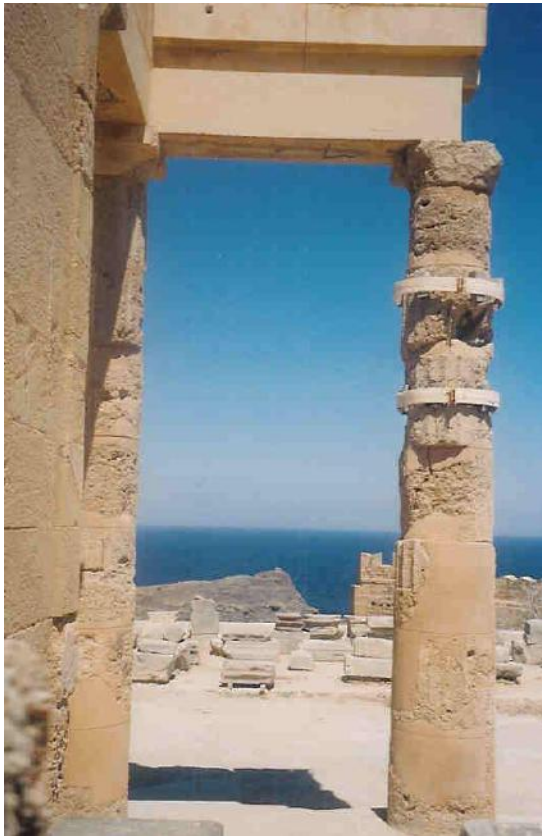
Figures 137a, b: a column of the transverse colonnade of the stoa that presents problems of structural stability (source: Vacharopoulou -- personal photographs, 2003).
