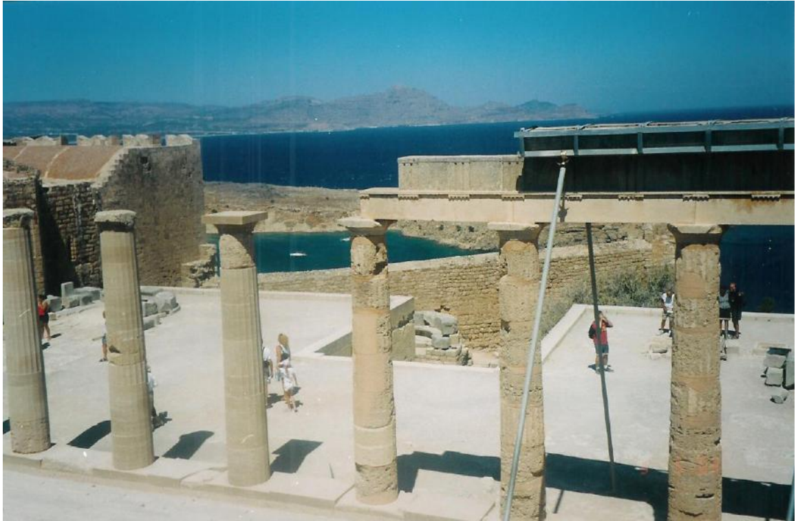
Figure 126: view of the restored transverse colonnade of the Stoa (source: Vacharopoulou -- personal photographs, 2003).
