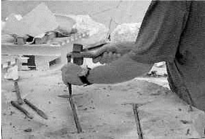
Figure 41a: removal of iron reinforcements by mechanical means (source: Maurommatis 2003, 28).
