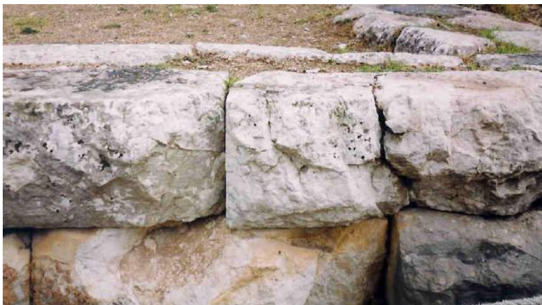
Figure 86c: restored stone members of the Gymnasium Propylon showing how surfaces will be protected by reassembly of old members and integration of new ones
