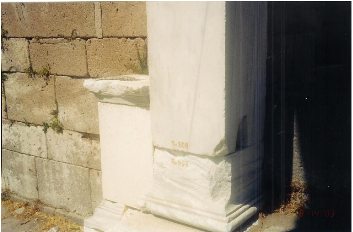
Figure 183b: integration of new and old members, leaving breaks and small defects visible and showing the inscription of the member number (source: Vacharopoulou -- personal photographs, 2003).
