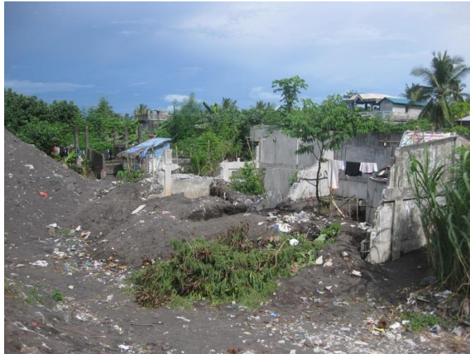
Figure 7.6 Ruined homes in Barangay Binitayan, which was downstream of barangays devastated by debris flows but was still devastated by hyperconcentrated flows and some boulder laden flows (September 2010). Source: author's own.
