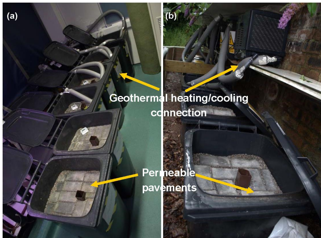
Figure 1. (a) Indoor (b) Outdoor experimental bins for Permeable Pavement Systems with combined PPS-GSHP.
