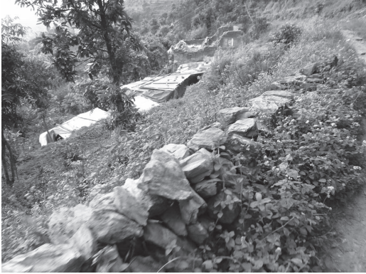
Photo 1 : Damaged house (back) and temporary hut (near) in Ahare. (August 2015)
