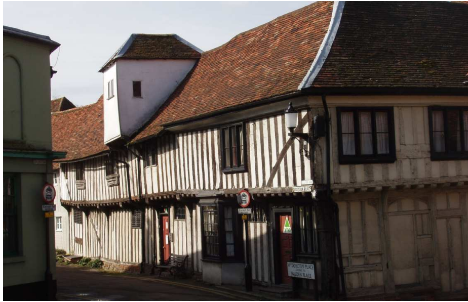
Photograph 5: A former malting on the corner of Middleton Place, now a private residence, once a saffron warehouse.
