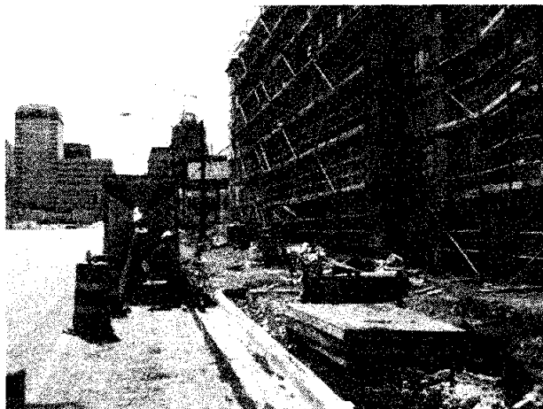
Figure 2. Picture of construction site scene.
