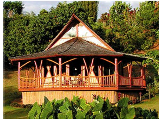
Gambar 2. 15. Bamboo Houses Stand up to Hurricanes
