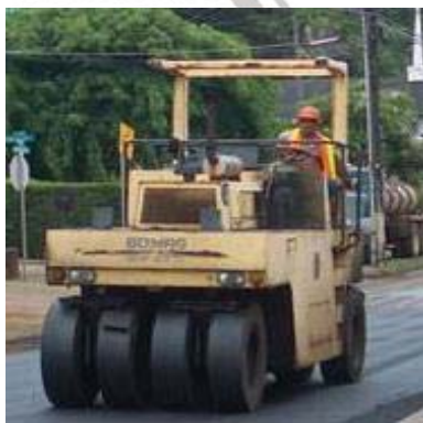
Gambar 2.2 Pneumatic rubber-tired rollers dan smooth-wheel roller
