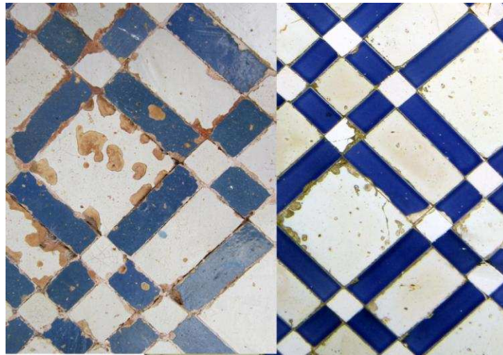
Fig. 3 - Moresque Blue 16 th century chess-like pattern (left side) compared to a cobalt blue 20 th century integration (right side) on the streets of Vila Viçosa
