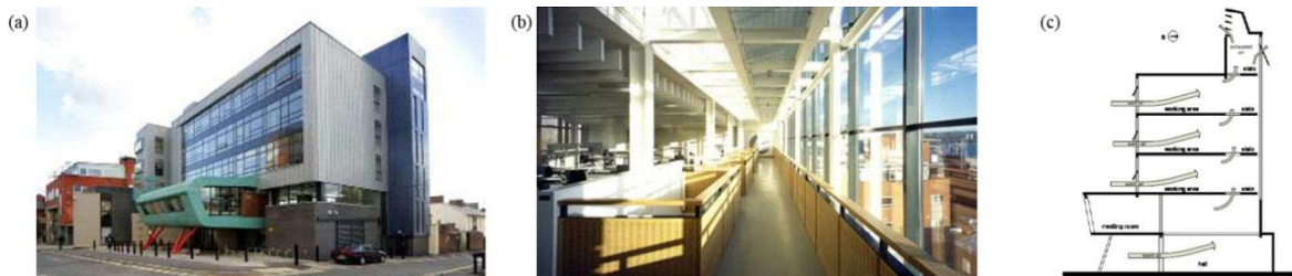
Figure 3. The ICoSS building study: (a) north-facing entrance view, (b) internal south-facing glazed façade, (c) section showing the natural ventilation scheme.
