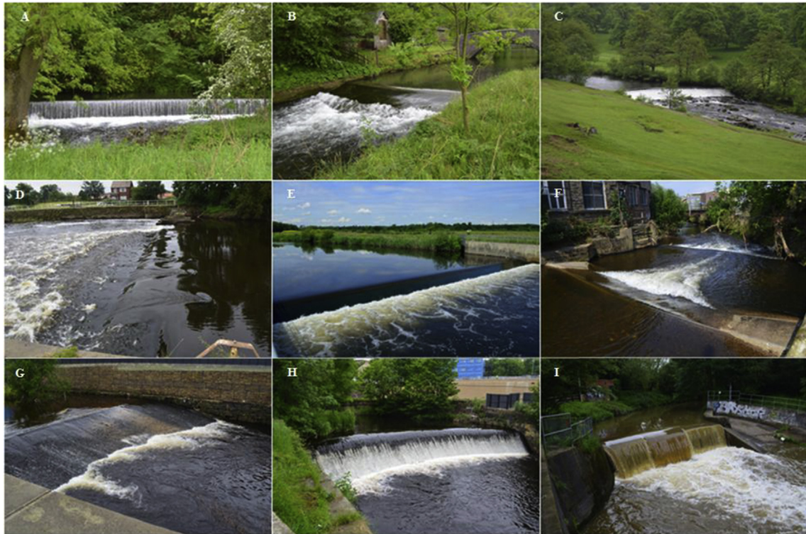
Fig. 1. Images of the nine main weir sites. Sites A, C, D, H and I are variations of Broad Crest Type; sites B and F are Flat V type and sites E and G are Crump type weirs.
