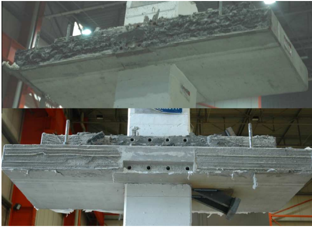
Fig. 14. Well executed and non satisfactory-filled joints as revealed at the demolition of the mock-up.
