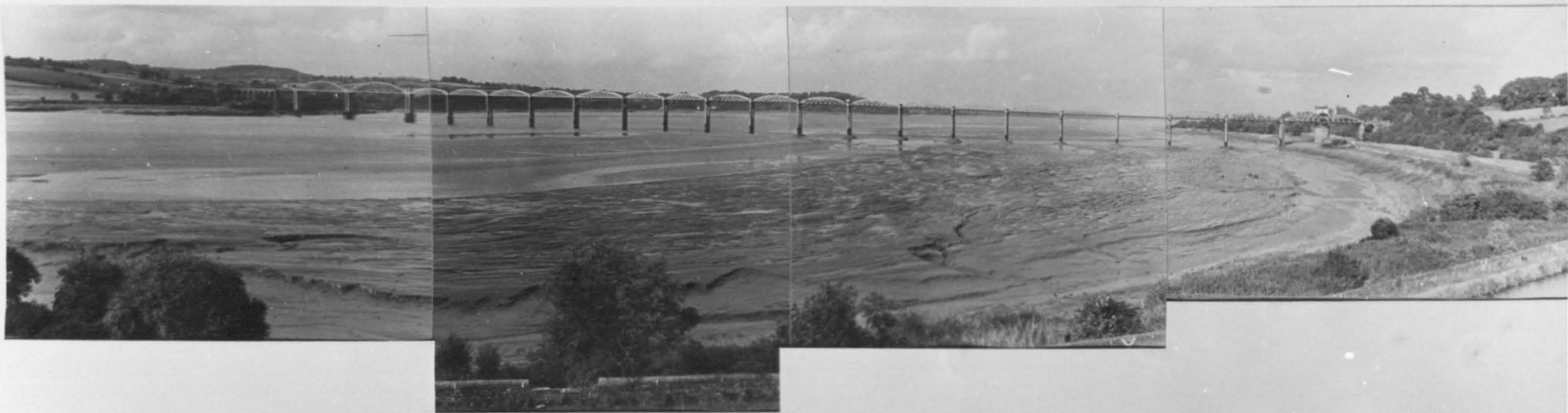
FIG. 4.2a VIEW OF SEVERN BRIDGE LOOKING N.E. FROM SHARPNESS.
