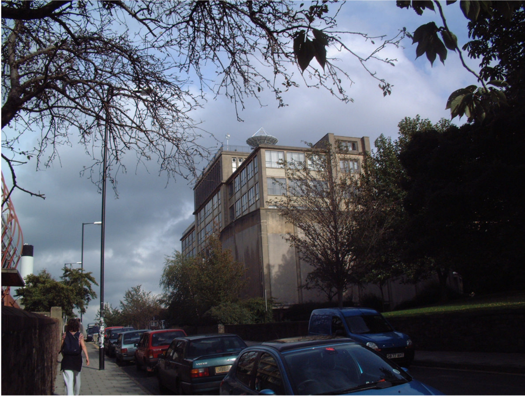
Figure 1: View towards Physics Building from Tyndall Avenue
