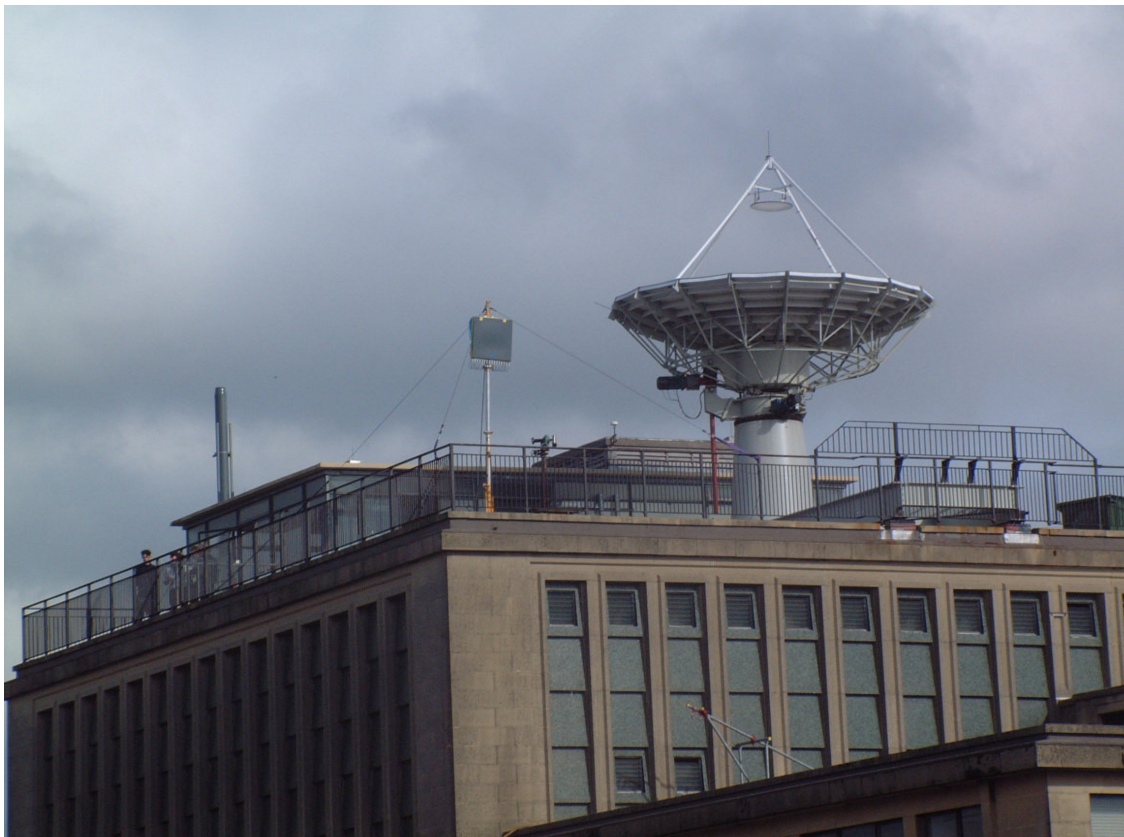
Figure 2: Array sighting on the roof of Physics Building.
