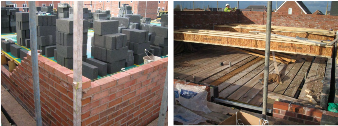
Figure 27 - Intermediate floor construction – external leaf built before inner leaf INAPPROPRIATE MATERIAL AND COMPONENT SELECTION
