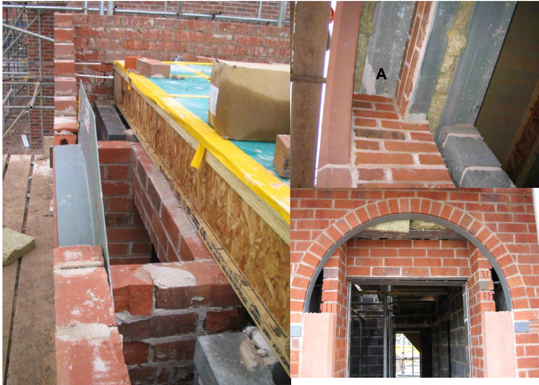
Figure 3 – Construction of recessed front door
