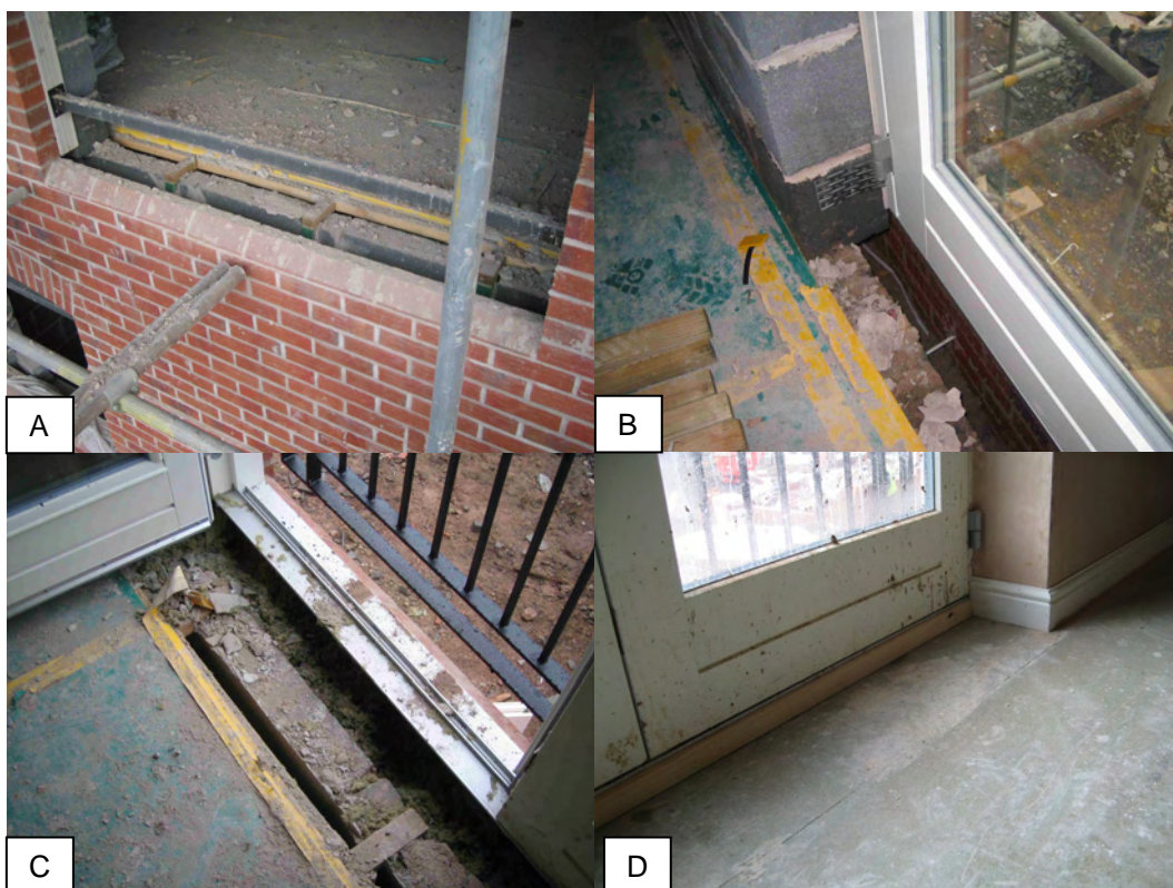
Figure 18 – Juliet balcony threshold in various stages of construction
