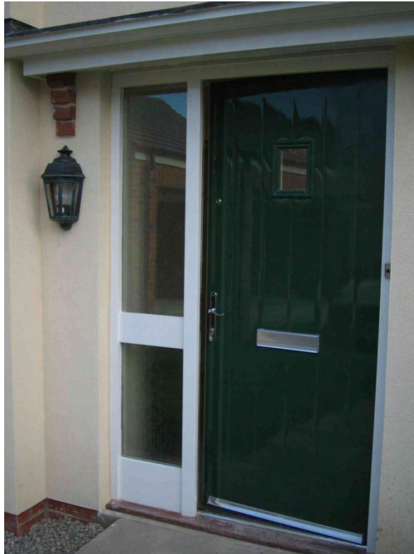
Figure 30 – New door and sidelight window
