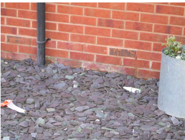
Figure 53 - Photograph and thermal image of external wall-ground junction (one of the first dwellings to be constructed showing thermal bridging at slab edge – see paragraph 64)
