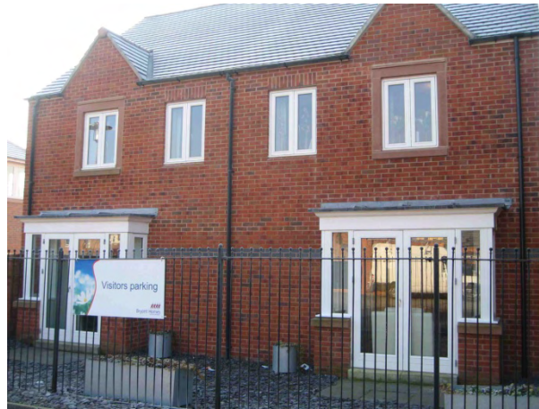
Figure 5 – Bay windows in completed dwellings
