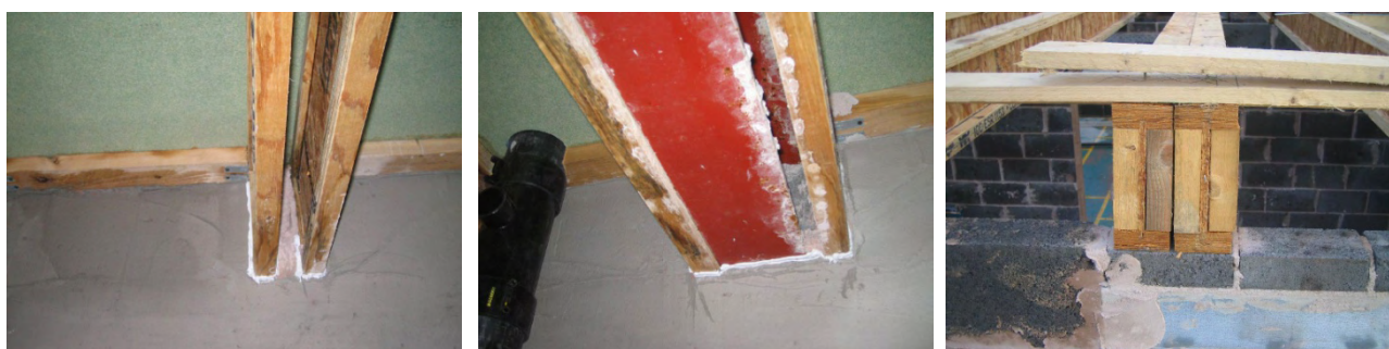
Figure 14 – Multiple adjacent built-in joists and beams
