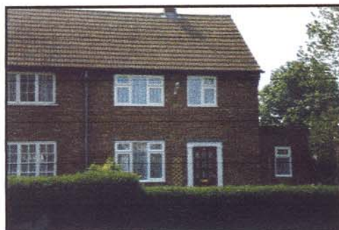
Chapelfield B from front. Note flue for wall mounted heater below living room window.
