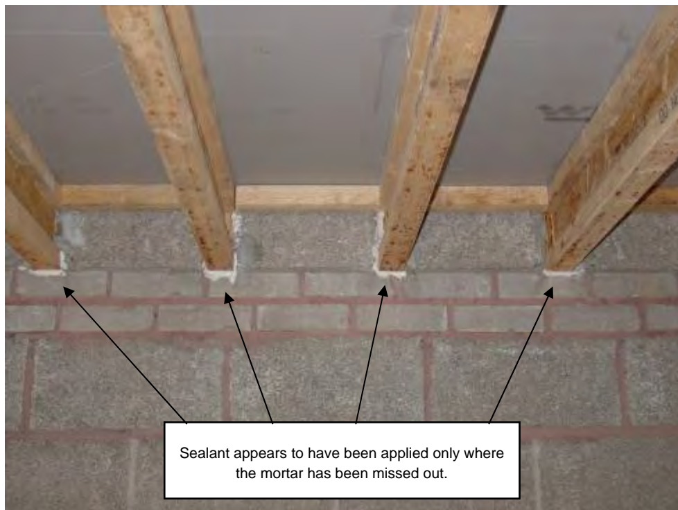
Figure 2 Partial application of mastic sealant (developer B).
