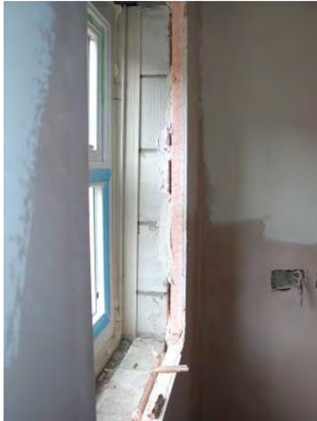
Figure 10 Discontinuous ribbons of adhesive around window opening.
