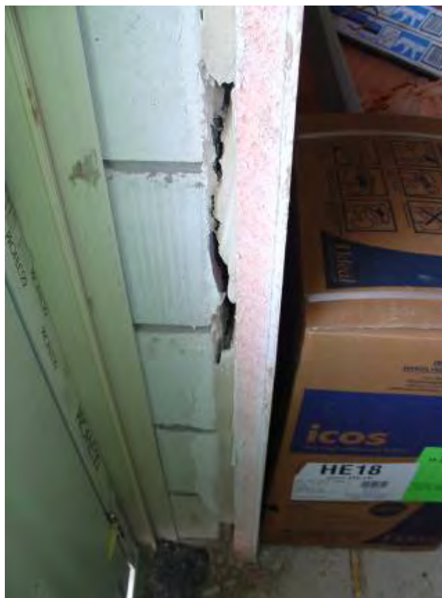
Figure 11 Discontinuous ribbons of adhesive around door opening.
