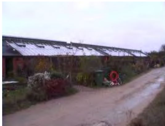
Figure 16 The Hockerton Housing Project.
