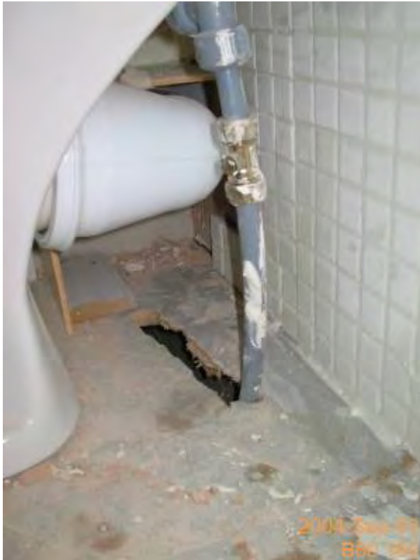
Figure 13 Unsealed service penetrations around WC.
