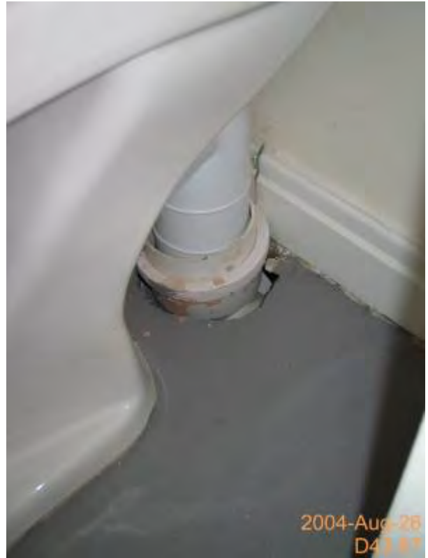
Figure 13 Unsealed service penetrations around WC.
