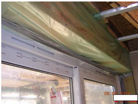
Figure 3.87 Air/vapour control layers not lapped to DPC 1 .
