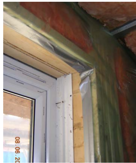
Figure 3.88 Vapour control layer returned in to reveals and window/door heads.
