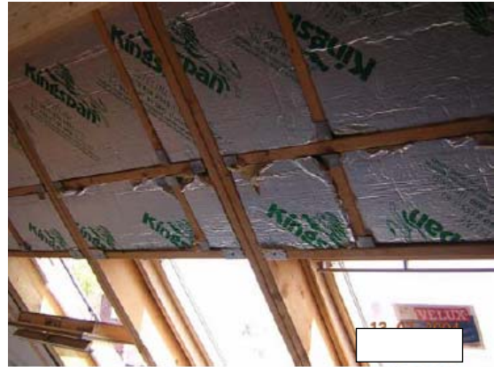
Figure 3.55 Insulation prior to fitting of insulated lining.
