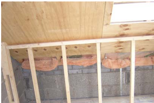
Figure 3.58 Cavity wall – roof junction.
