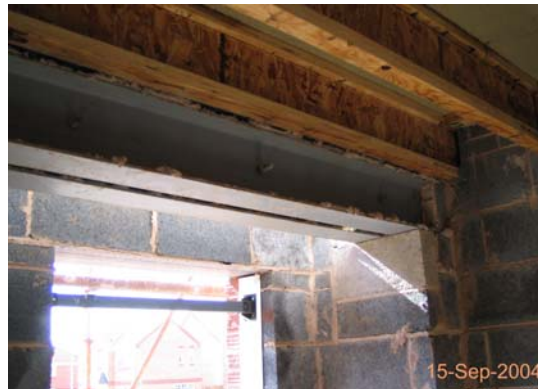
Figure 3.71 Steel work at large openings.
