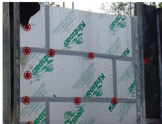
Figure 3.90 Fixing and sealing of partial cavity wall insulation in masonry construction.
