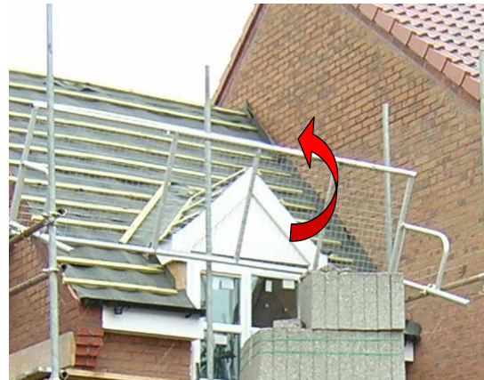
Figure 3.53 Gap in insulation adjacent to gable wall and structural thermal bridge (arrows).
