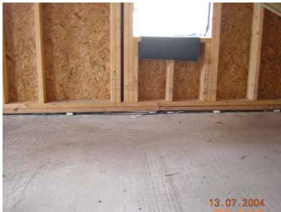
Figures 3.14 and 3.15 Plastic spacers used to level timber frame.
