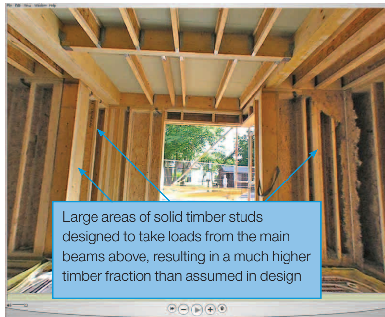
Figure 10: Screen capture from panoramic of gable wall section in House F
