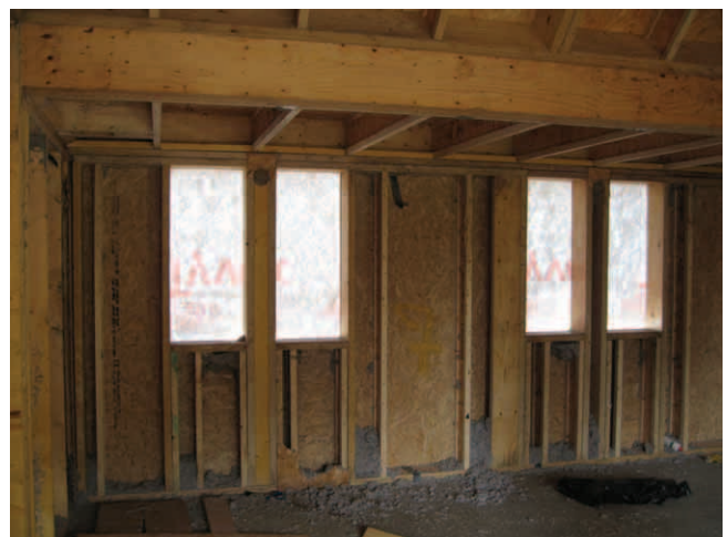
Internal panel structure showing additional timber, particularly around openings
