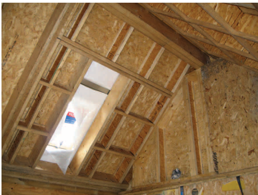
Figure 11: Additional timbers in roof panels
