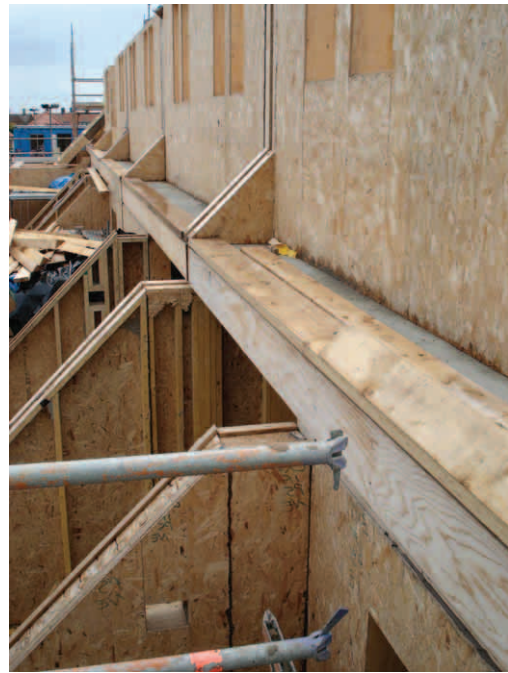
Junction under construction
