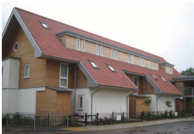
Figure 3: Elm Tree Mews – completed scheme
