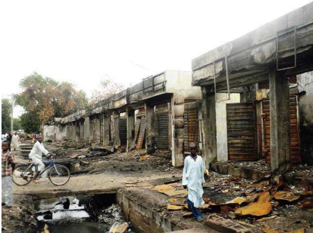
Burnt properties: Houses and shops burnt by operatives of the joint military task force (JTF) at Budun area of Maiduguri. The area was suspected to be a stronghold of Boko Haram (photo by Hamza Idris).
