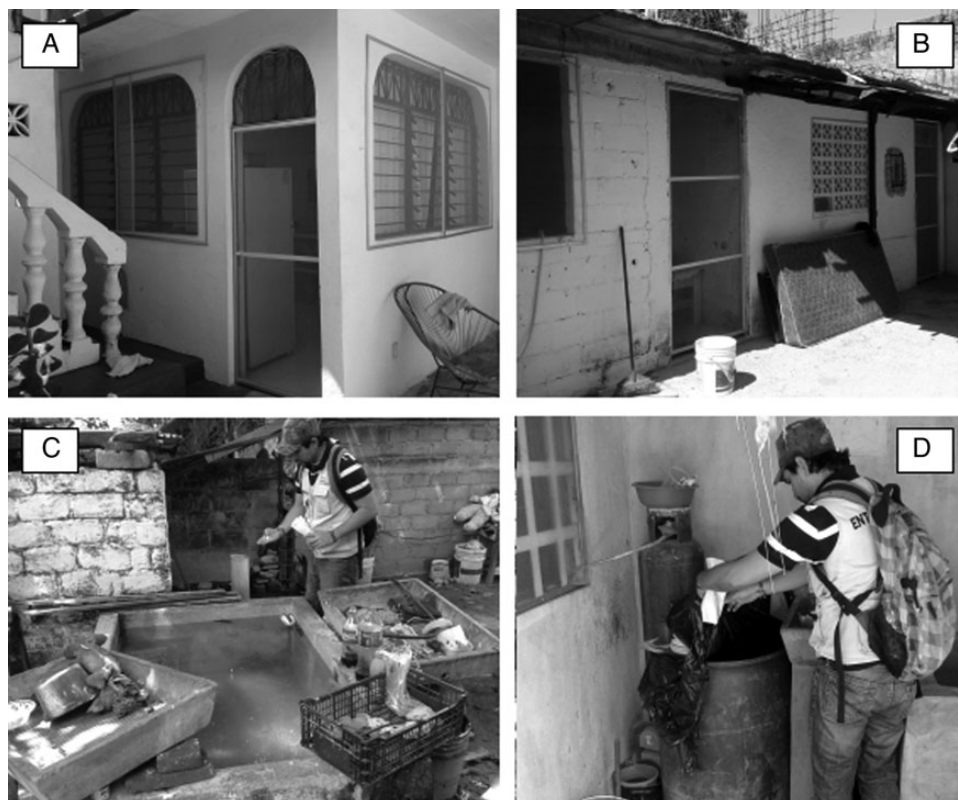
Figure 2. Photographs show (A,B) the long-lasting insecticidal net screens ([LLIS]; Duranet ® [Clarke Mosquito Control, Roselle, IL, USA]) mounted on aluminum frames and fixed to windows and external doors of treated houses and (C,D) the targeted treatment (TT) of the most productive Aedes aegypti breeding sites with the larvicide Natular ® DT (Spinosad 7.48%) in Acapulco Mexico.
