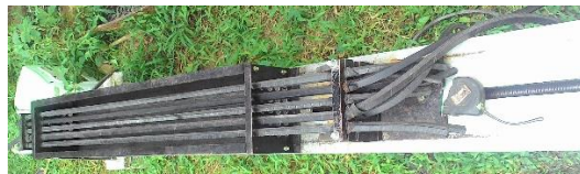
b. Installation of the waste tire on the second clamp
