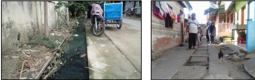
Figure 3. Drainage condition at four hamlets (Source: Observation)
