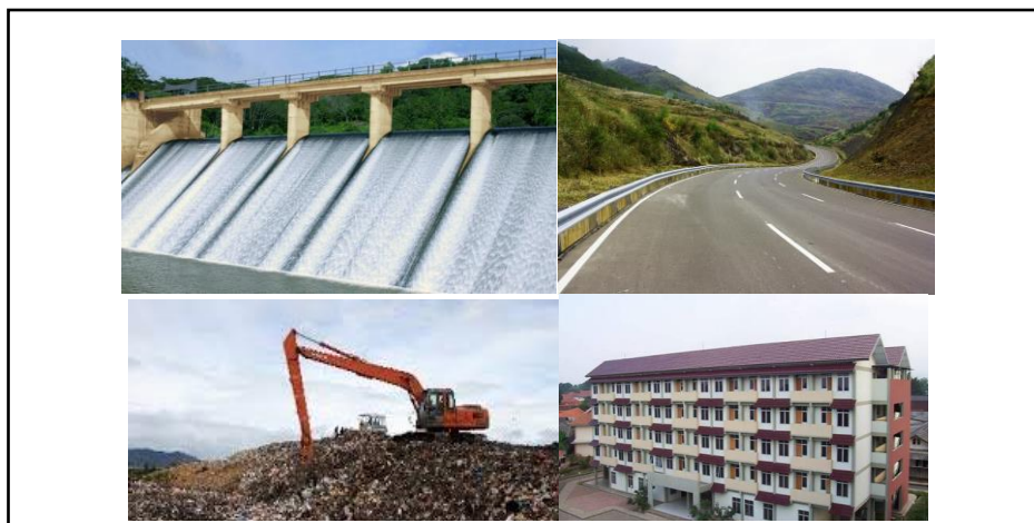
Figure 1. Example of Public Works Land Public Housing Infrastructure
