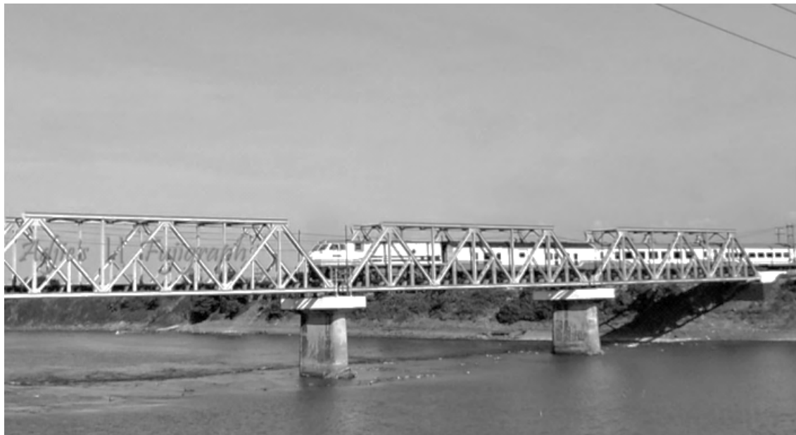
Figure 1. Porong Steel-truss Railway Bridge (Source: www.skyscrapercity.com)
