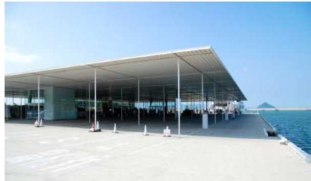
Figura 33. Naoshima Ferry Terminal.
