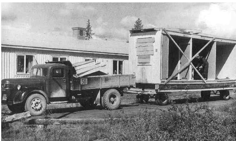
Fig. 27. Transportation of some modules for the assembly of a skivhus . K. Lindbäk, 1962
