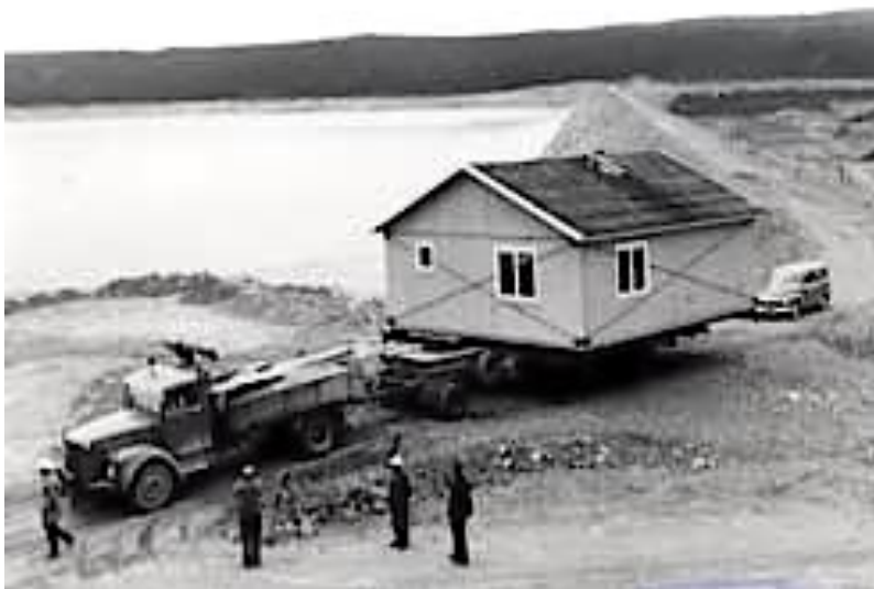
Fig. 50. House being moved from Messaure. J. Palmqvist Fig. 51. Same house, on its way to Jokkmokk. J. Palmqvist
