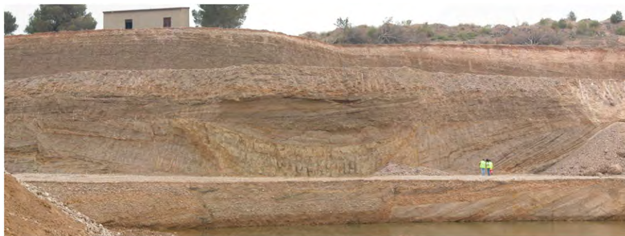
FIGURE 10 Slow subsidence and later sudden-collapse case analysed in Example 6, SW Garrapinillos Village. Dissolution of Neogene caused subsidence in fluvial deposits and development of fractures and faults. A collapse is developed in the central area, where mud settled out. Deformation is attenuated to the top and new gravel beds cover the previous feature [Colour figure can be viewed at wileyonlinelibrary.com ]
