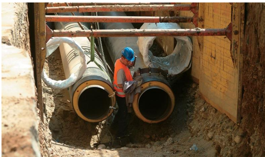
Figure 2.2: Preinsulated district heating pipes installed underground (Danfoss, 2015)
