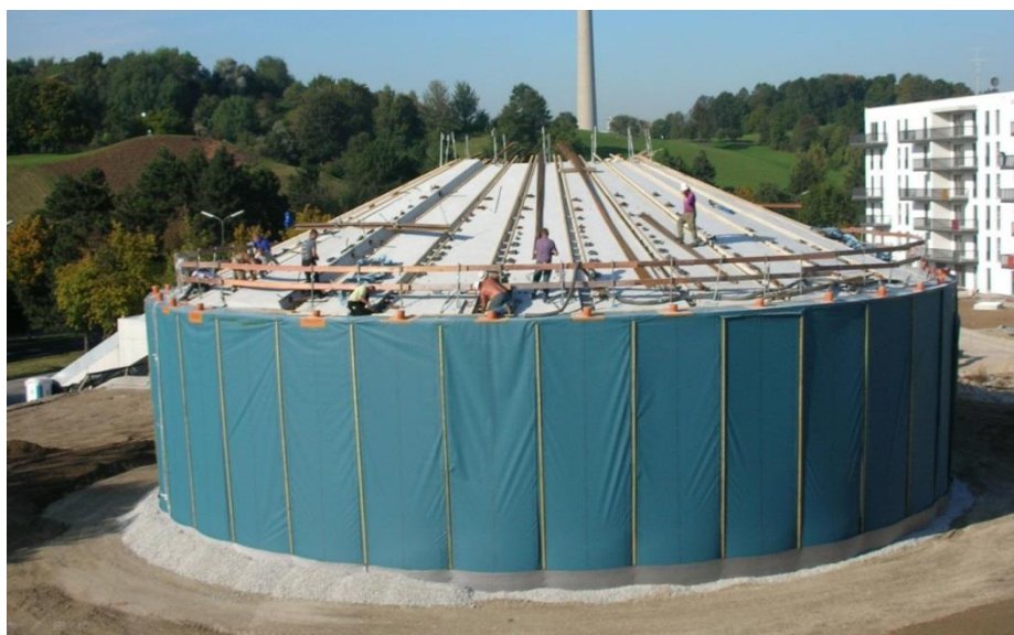
Figure 2.12: Construction of hot water tank (Solites, 2014a)
