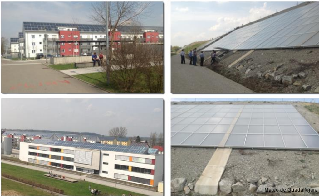
Figure 2.19: Solar collectors integrated in the community of Crailsheim
