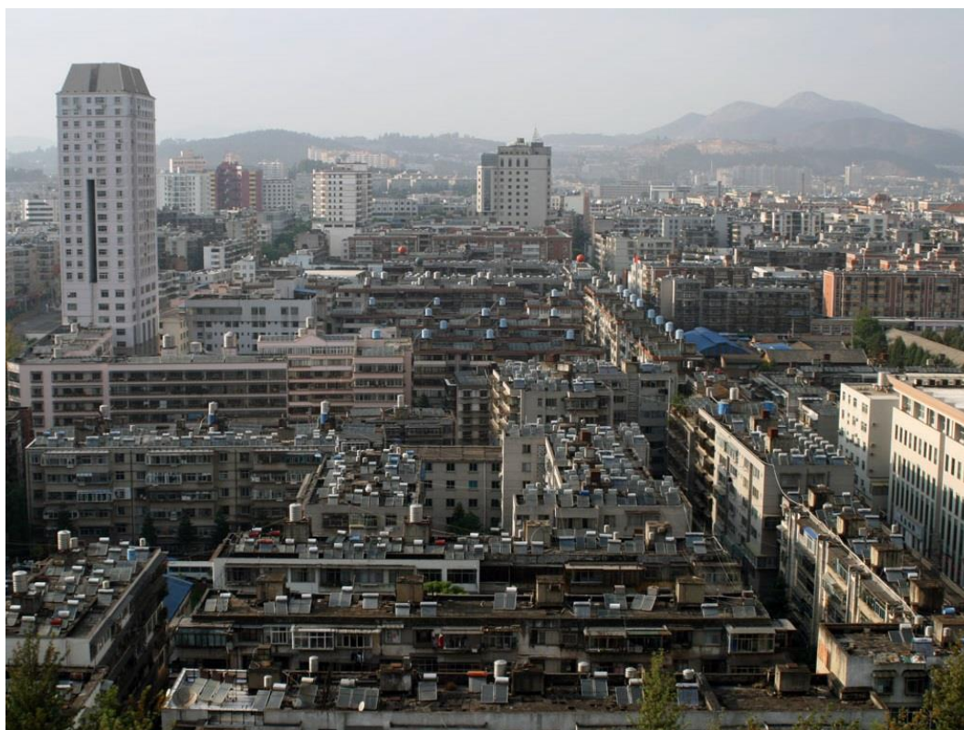
Figure 5.1: Solar water heaters installed in Kunming China
