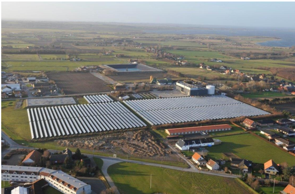
Figure 2.16: Solar thermal plant in Marstal (Sunstore-4, 2014)
