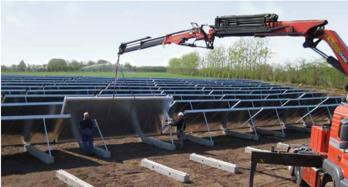
Figure 2.10: Flat plate collector installation (Arcon, 2014)
