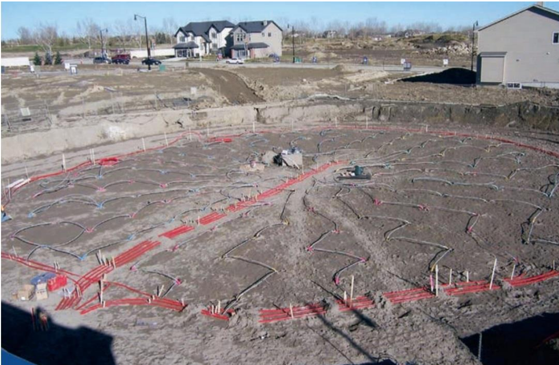
Figure 2.14: Drake Landing Solar Community borehole construction (canmet ENERGY, 2015)
