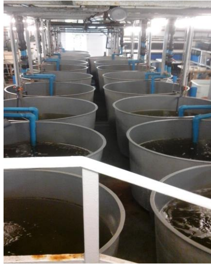
Figure 7: The fiberglass tanks of line 1 of the laboratory of aquaculture.
