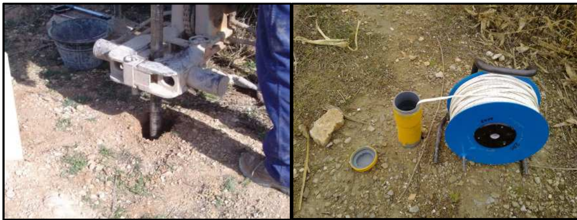
Fig. 3-4. Piezometers drilling and depth to groundwater monitoring.
