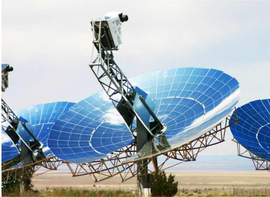
Figura 25 Sistema disco-Stirling SunCatcher™ de SES [25].
