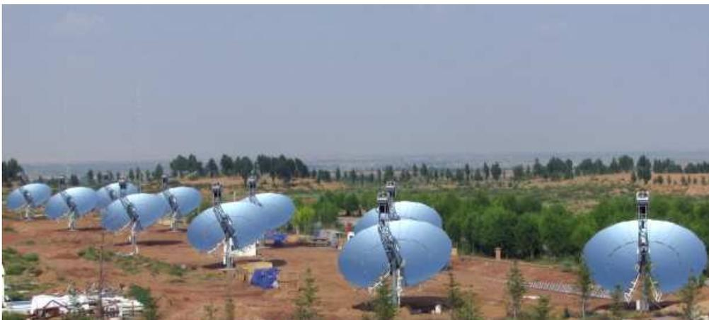
Figura 21 Parque solar de disco-Stirling Cleanergy [30].
