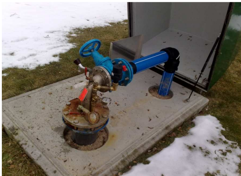
figure 2.4 shows the water intake and well house 80.217.
