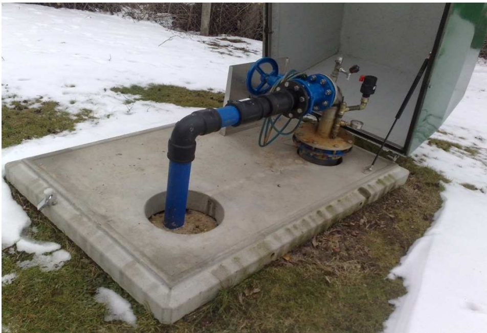
figure 2.2 shows the water intake and well house 80.321.
