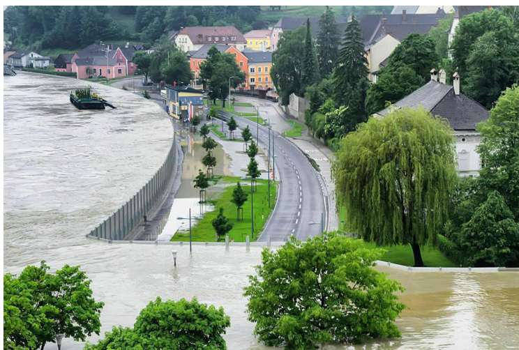
Figure 5. Mobile flood walls in the city of Grein, further downstream of the river basin Eferding. Only a couple of centimeters between the top of the flood walls and the water level (Source: Ariva.de)
