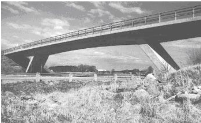
Figur 7 Snedbening, balkbro (Vägverket (c), 2009)
