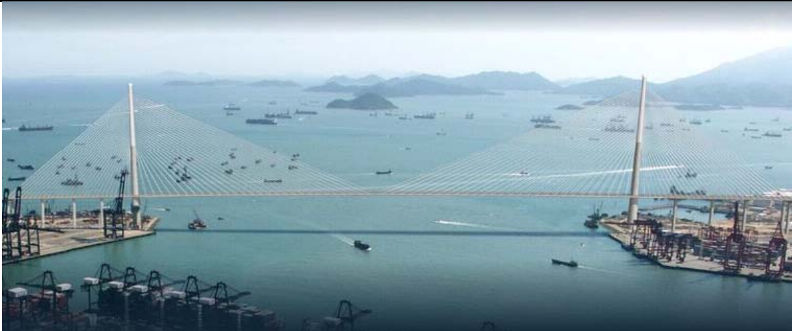
Figur 14 Stonecutters Bridge, Hongkong, spännvidd 1018 meter (Highway department, Hong Kong, 2009)
