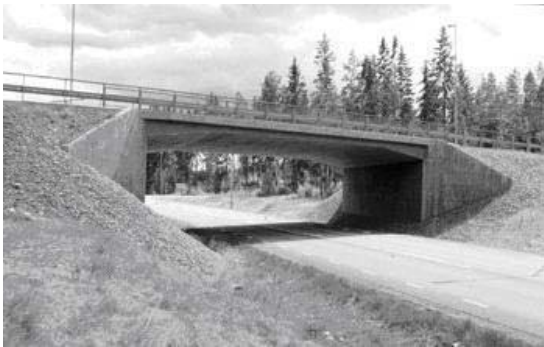
Figur 4 Plattrambro (Vägverket (c), 2009)
