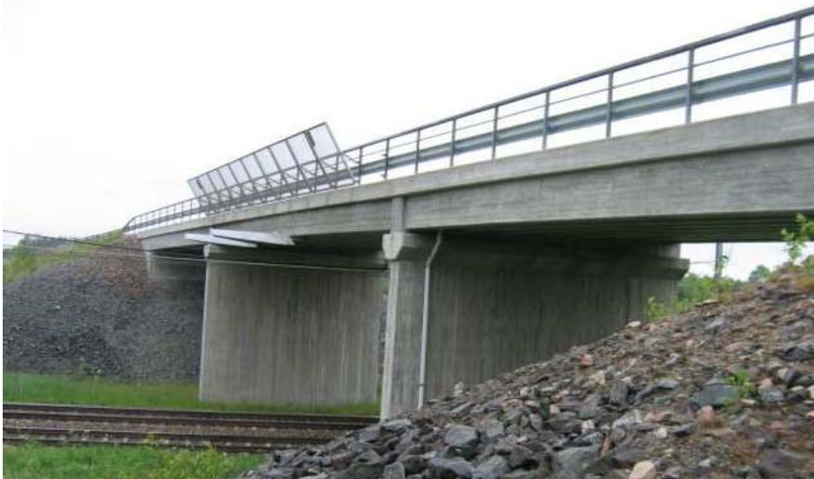
Figur 22 NCC Montagebro, 3-fack (NCC (c), 2009)
