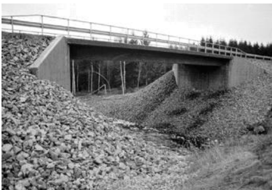
Figur 5 Balkrambro (Vägverket (c), 2009)
